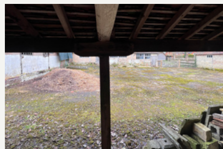
3. NORTH - VIEW FROM BYRE
