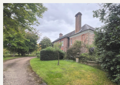
5. DRIVE ALONG WEST ELEVATION
