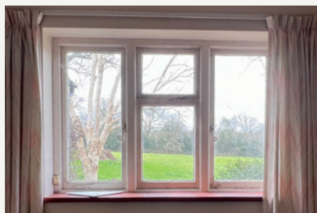
4. WEST - COTTAGE VIEW TO FIELD
