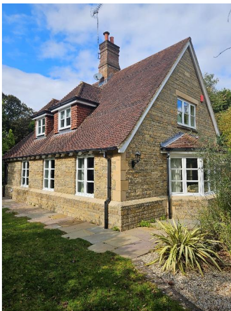
View looking north west
