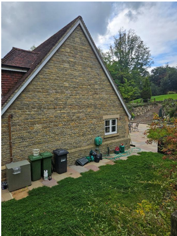
Side elevation facing north
