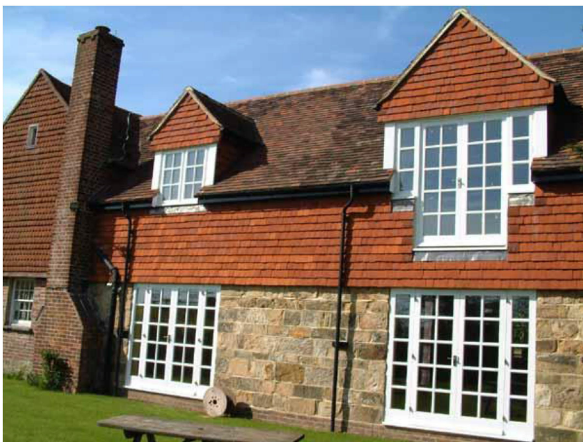
Fig 6: Example use of Aldershaw tiles, with 'restoration red' hung tiles, and 'dark antique' roof tiles.
