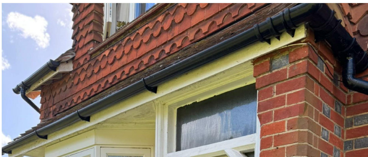
Fig 8: Existing black plastic gutters and downpipes.
