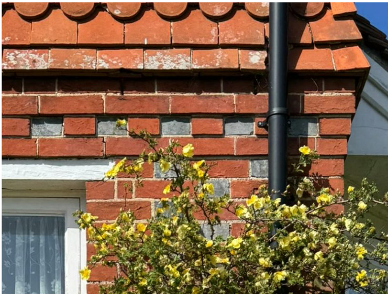
Fig 1: South-east corner, brickwork dentil.
