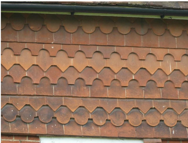
Fig 3: Hung tiles, with club, arrow, fishtail, and straight edge profiles.
