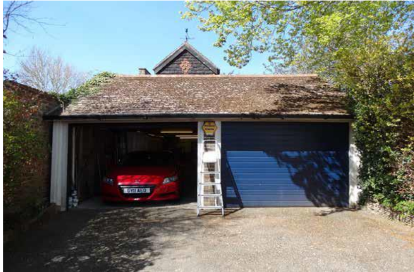
The Garage Frontage
