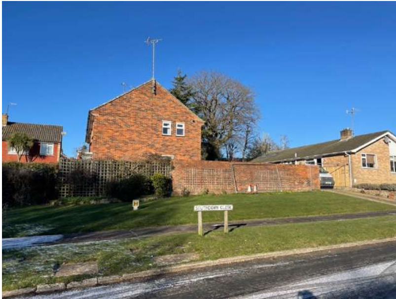
View looking north-west showing side elevation incl. driveway at the rear
