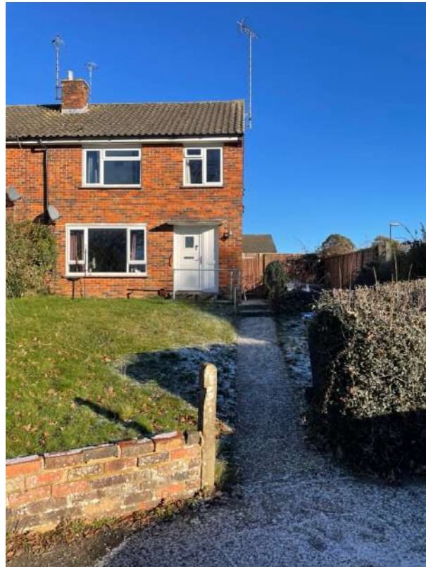
View looking north-east showing front elevation
