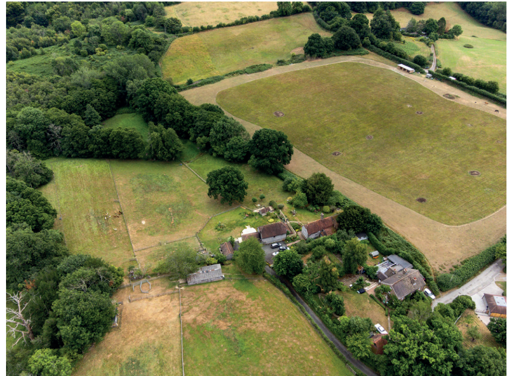
4. Drone view of Grove farm looking east (prior to repair work and enactment of DM/221393)
