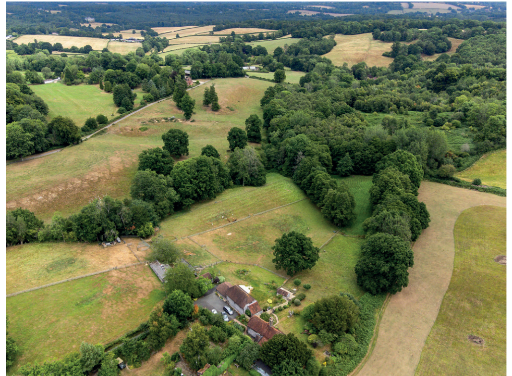
5. Drone view of Grove farm looking north (prior to repair work and enactment of DM/221393)
