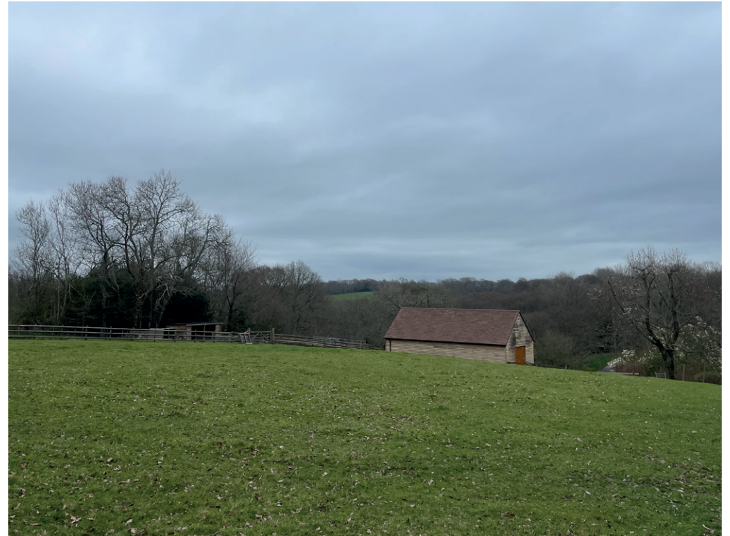
3. View of existing outbuilding
