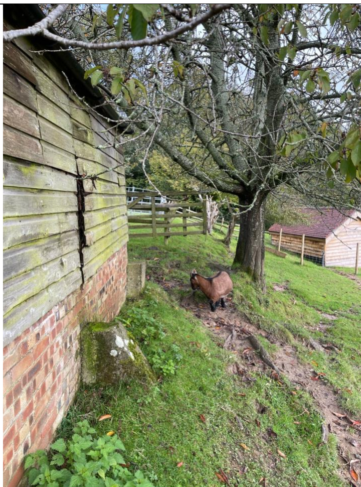
Photograph 4: Building B1 external and cherry tree.
