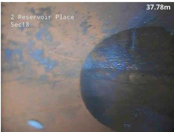
5, 00:02:53, 37.90 m Finish node, major connection without manhole, reference: Sewer
