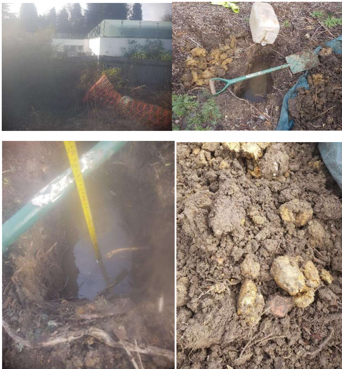
Fig 5. Soakaway test (site photographs)
