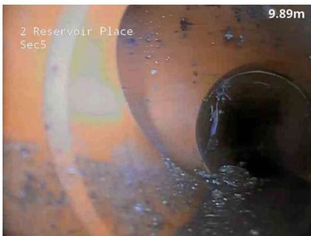
5, 00:00:48, 9.90 m Junction at 9 o'clock, 100mm dia
