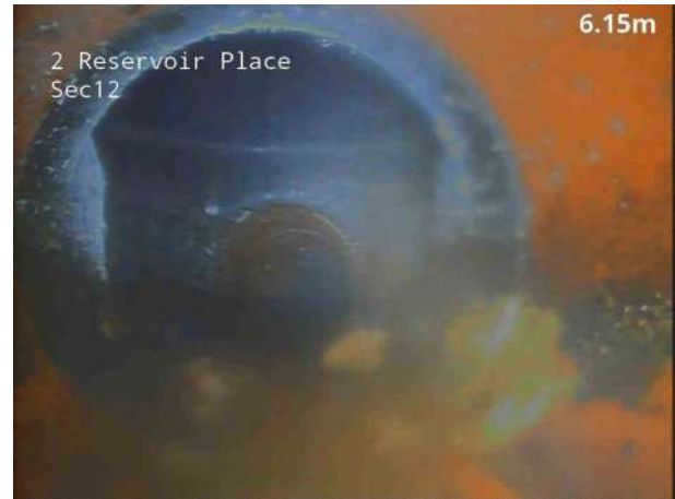
2, 00:01:44, 6.20 m Finish node, manhole, reference: MH5
