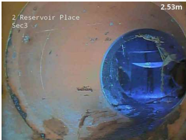
3, 00:00:32, 2.60 m Finish node, manhole, reference: MH8
