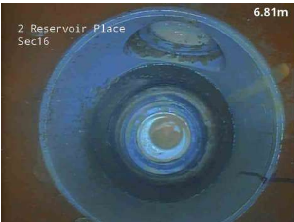
5, 00:00:41, 6.90 m Finish node, manhole, reference: FP
