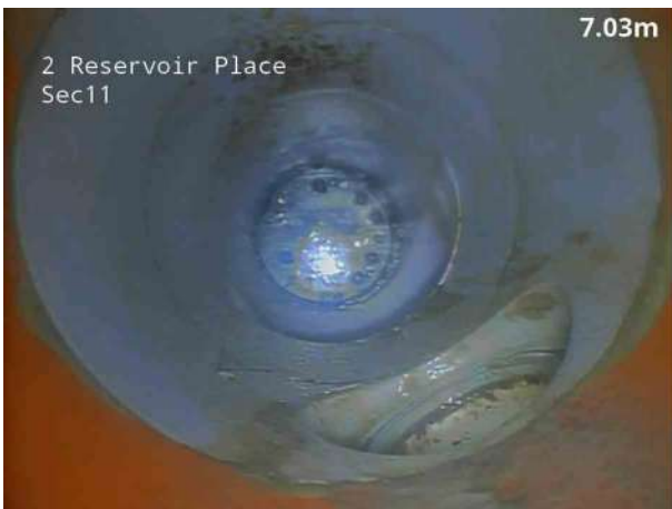
5, 00:00:27, 7.10 m Finish node, manhole, reference: SS2
