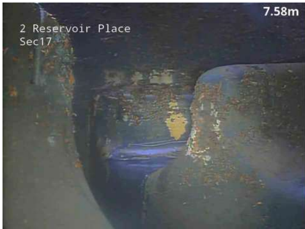
3, 00:00:36, 7.60 m Finish node, manhole, reference: MH2
