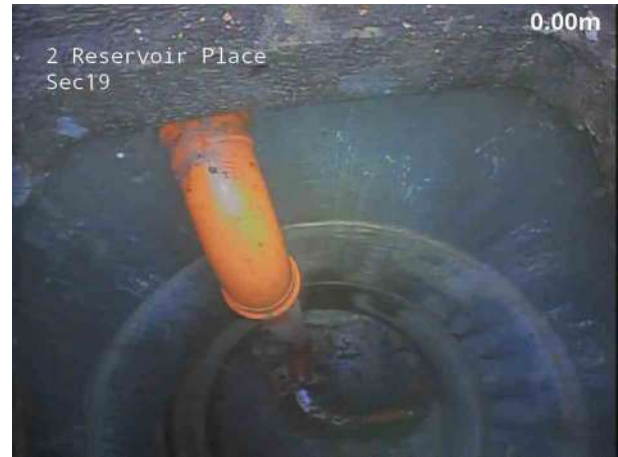
2, 00:00:09, 0.00 m Finish node, manhole, reference: FP
