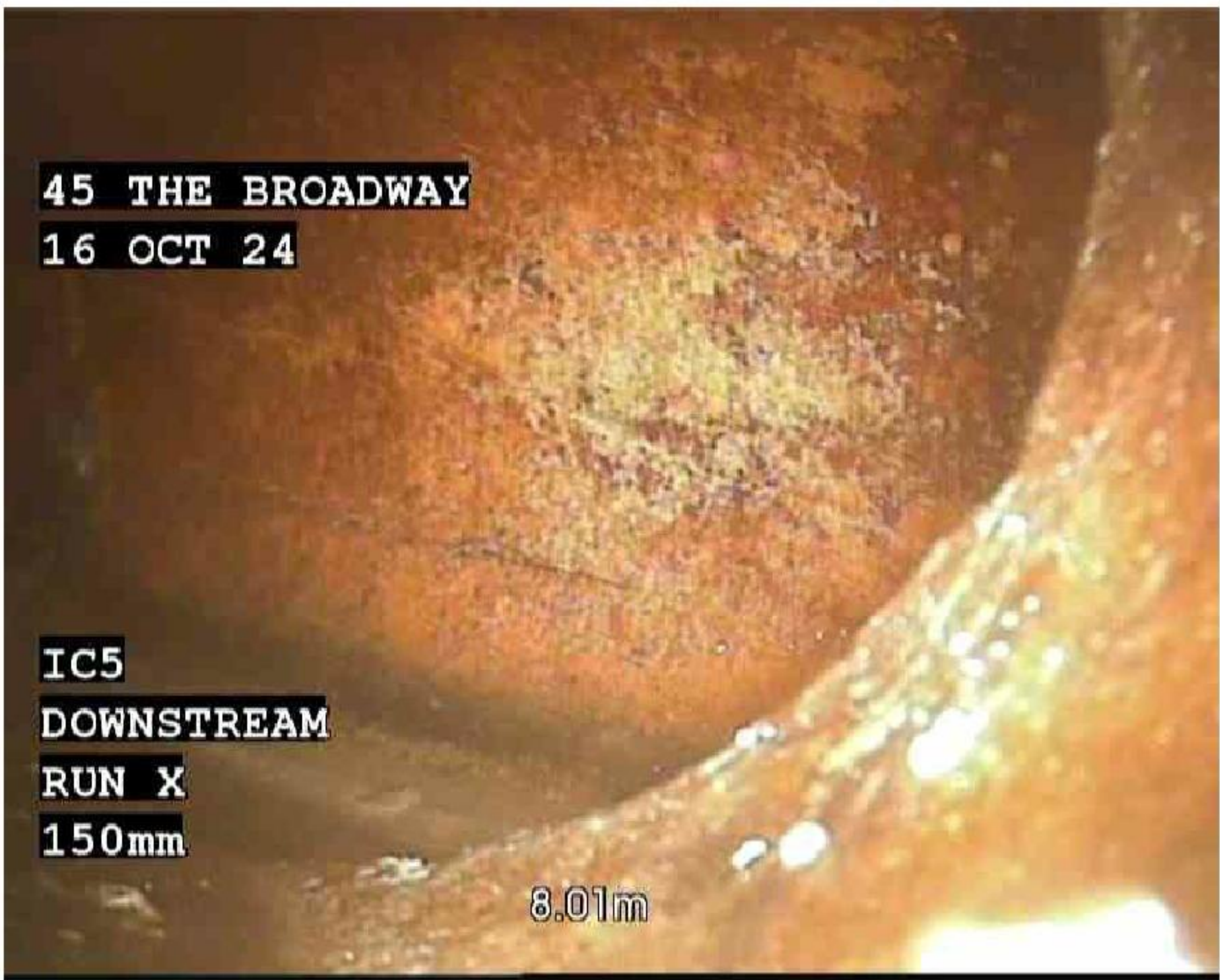
2, 00:00:44, 8.01 m Finish node, major connection without manhole, reference: RUN X, At saddle connection
