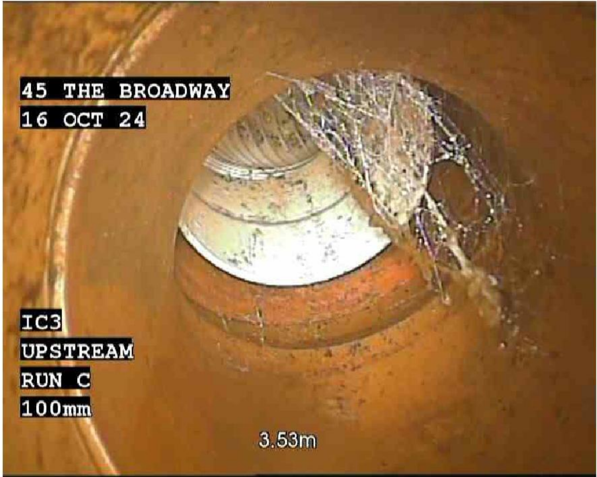
1, 00:00:16, 3.53 m Finish node, manhole, reference: IC3-C, At wc
