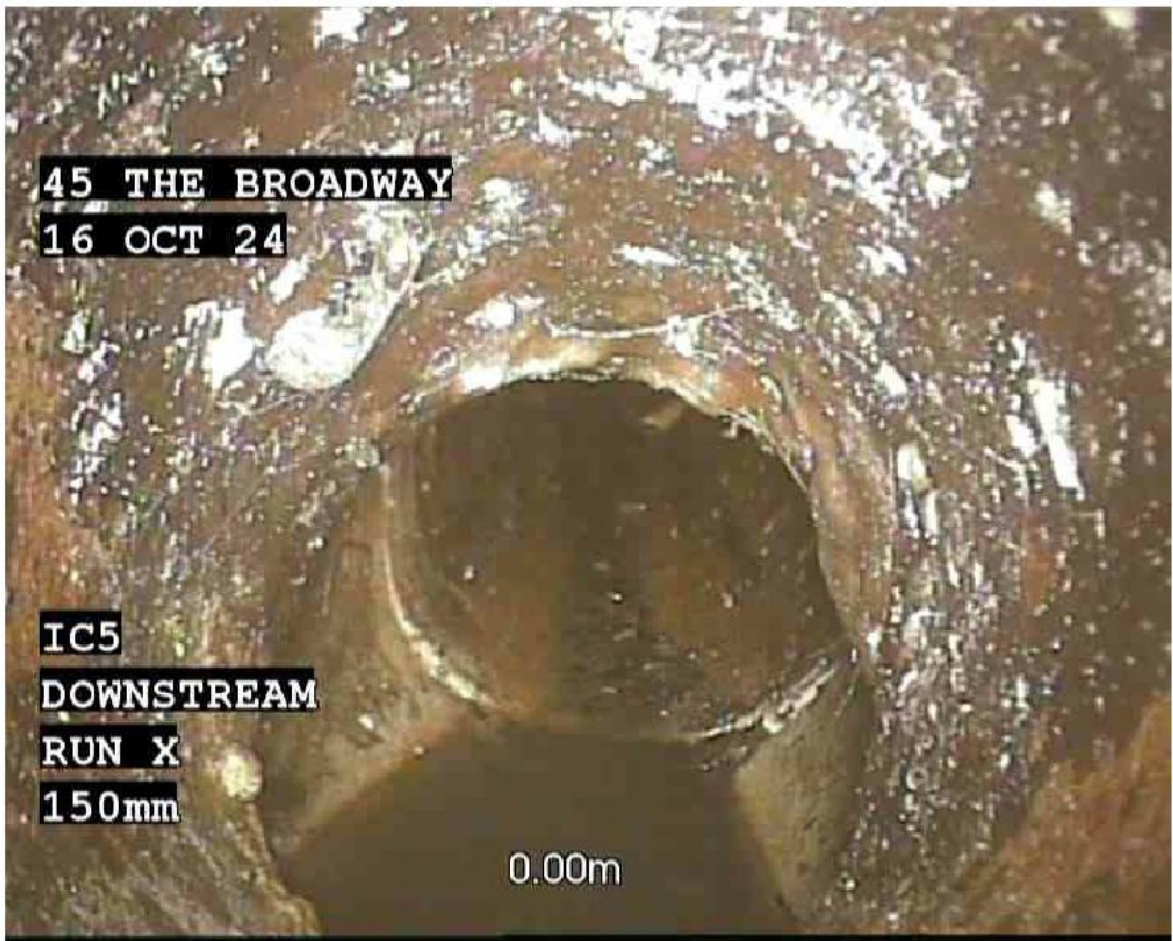
1, 00:00:00, 0.00 m Junction at 6 o'clock, 150mm dia, Interceptor trap
