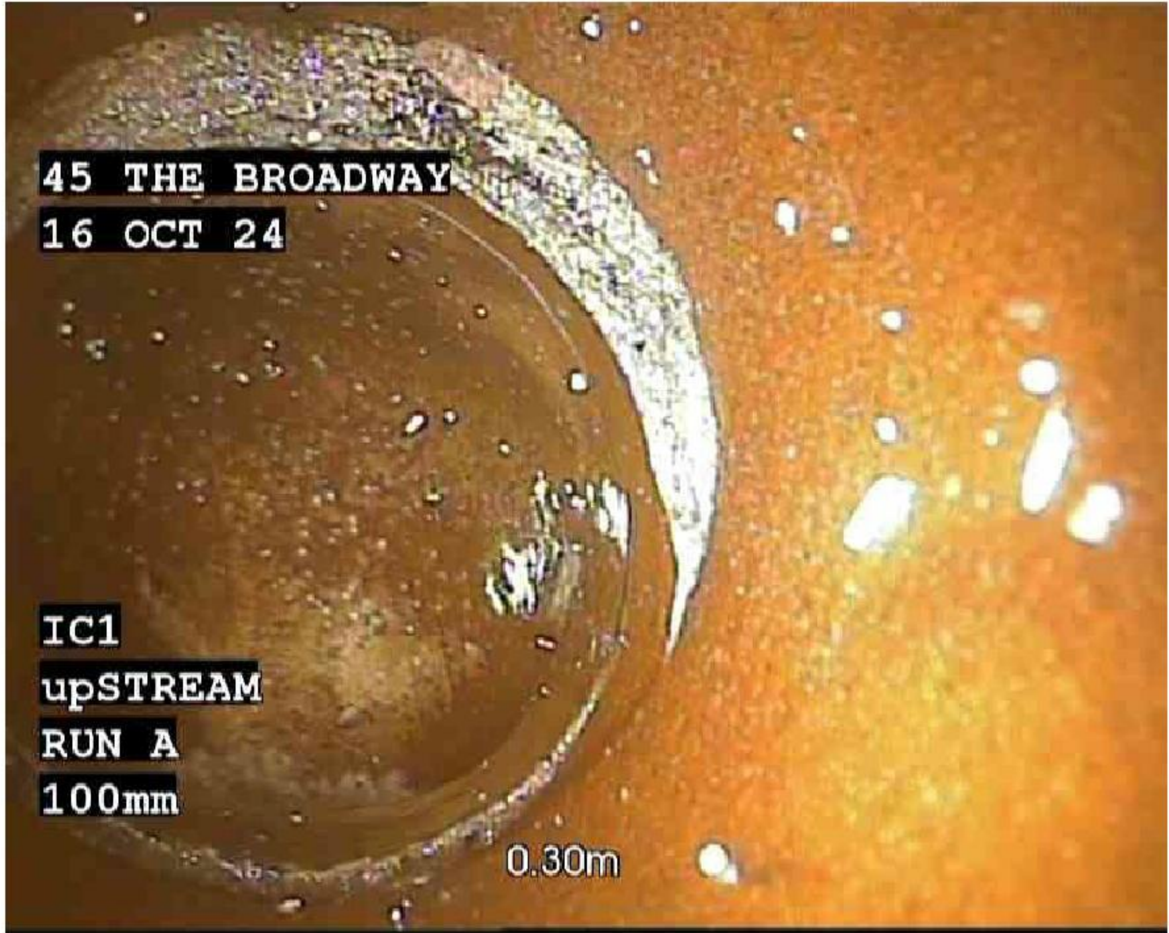
1, 00:00:02, 0.00 m Water level, 5% of the vertical dimension
