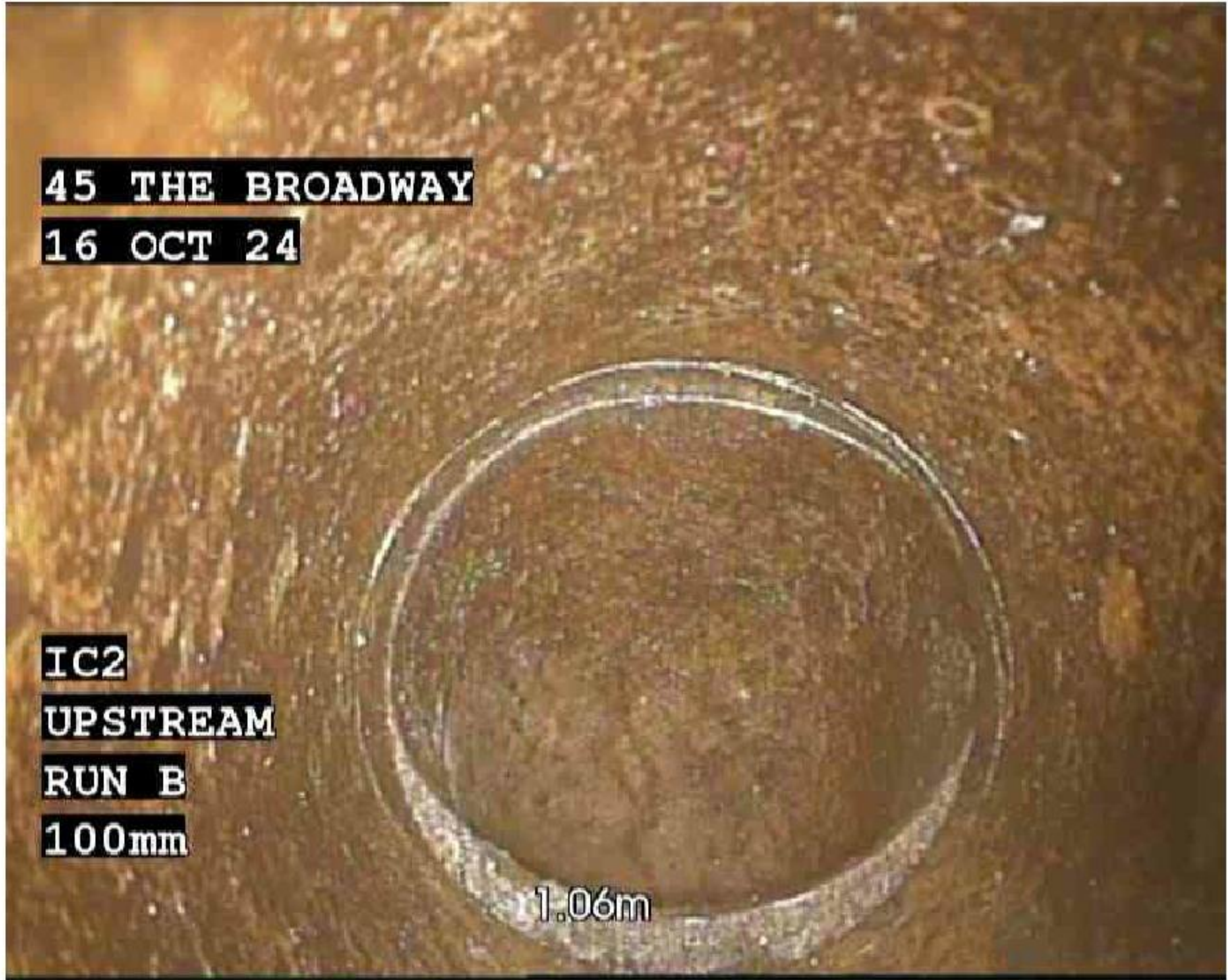
1, 00:00:12, 1.06 m Finish node, manhole, reference: IC2-B, At unknown gully assumed to be redundant
