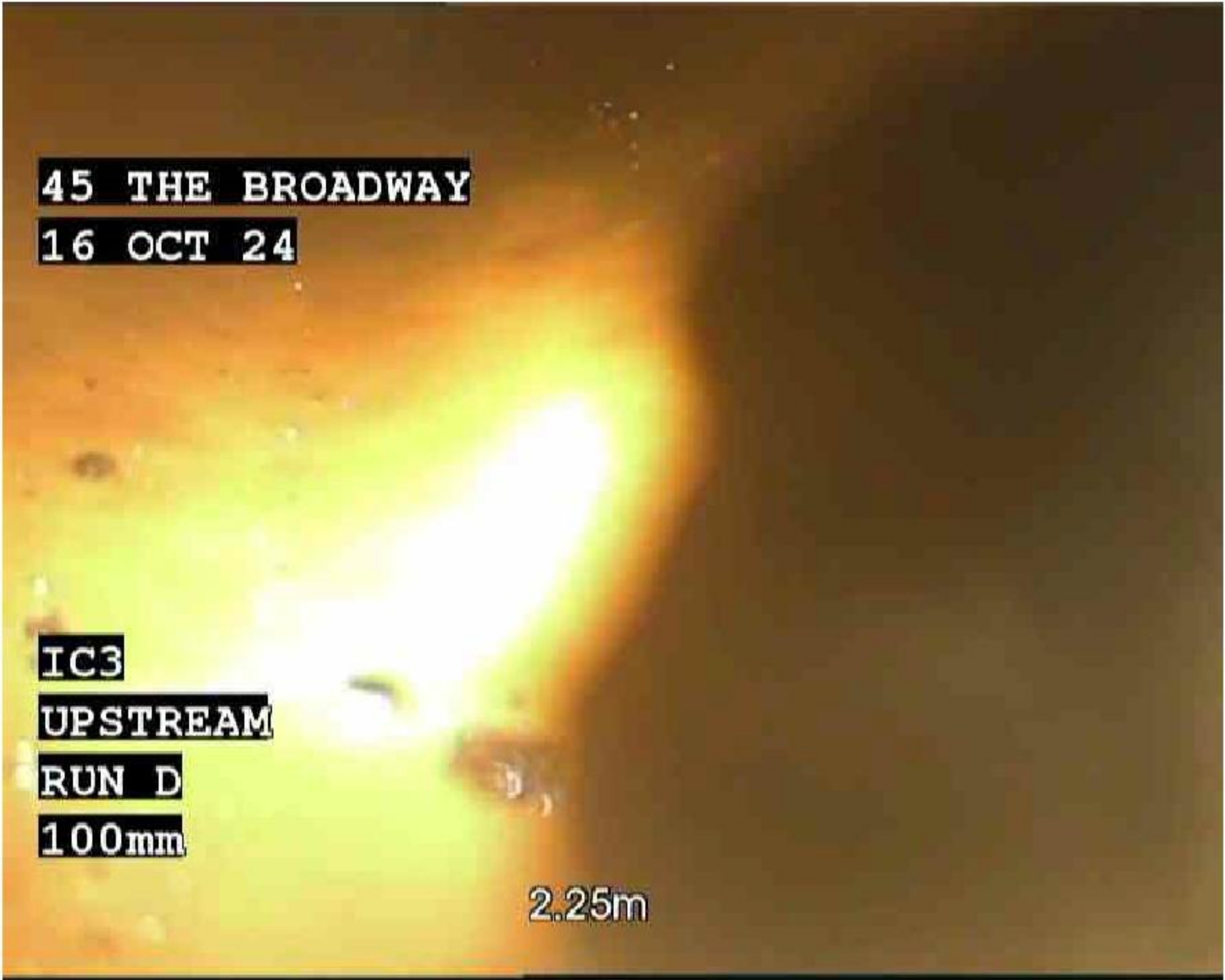
1, 00:00:20, 2.25 m Finish node, manhole, reference: At soil pipe
