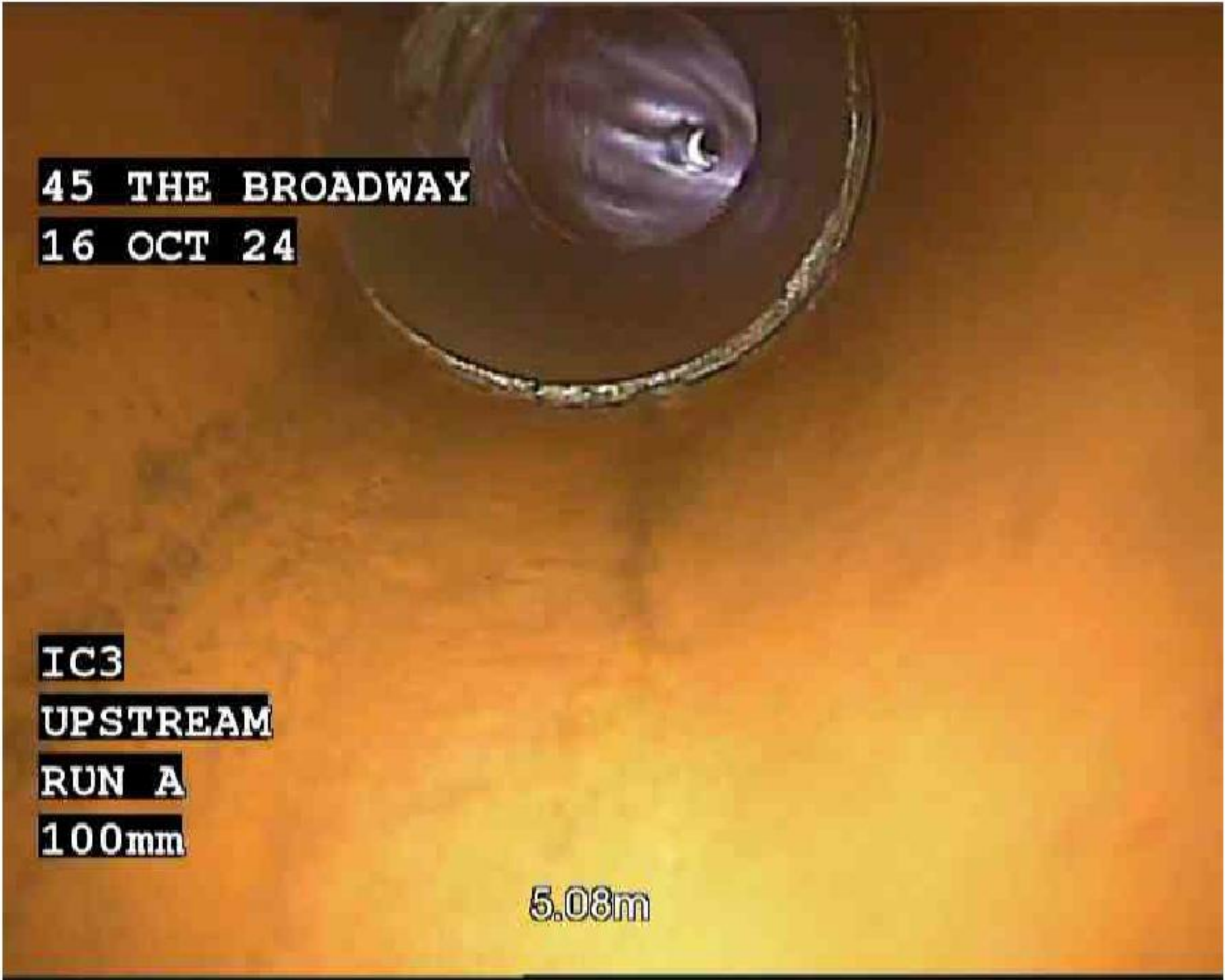
1, 00:00:42, 5.08 m Finish node, manhole, reference: IC3-A, At svp
