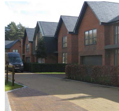
Block paving to shared surfaces and parking bays
