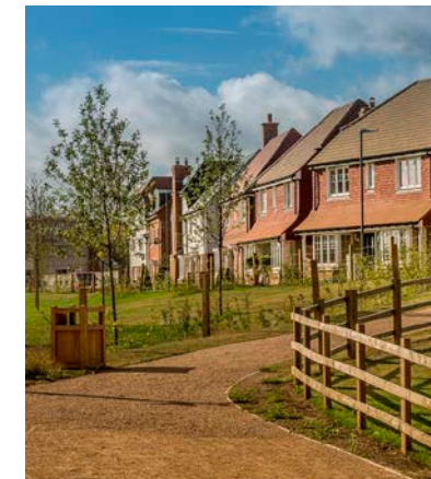
Hoggin gravel footways
