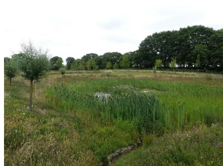
Landscaped attenuation basin
