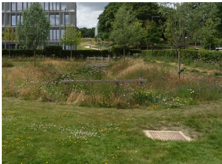
Landscaped attenuation basin
