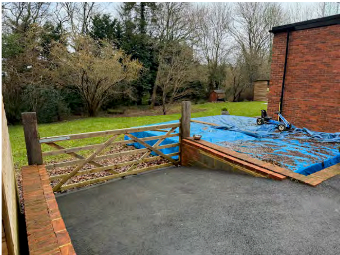
Facing northeast across garden
