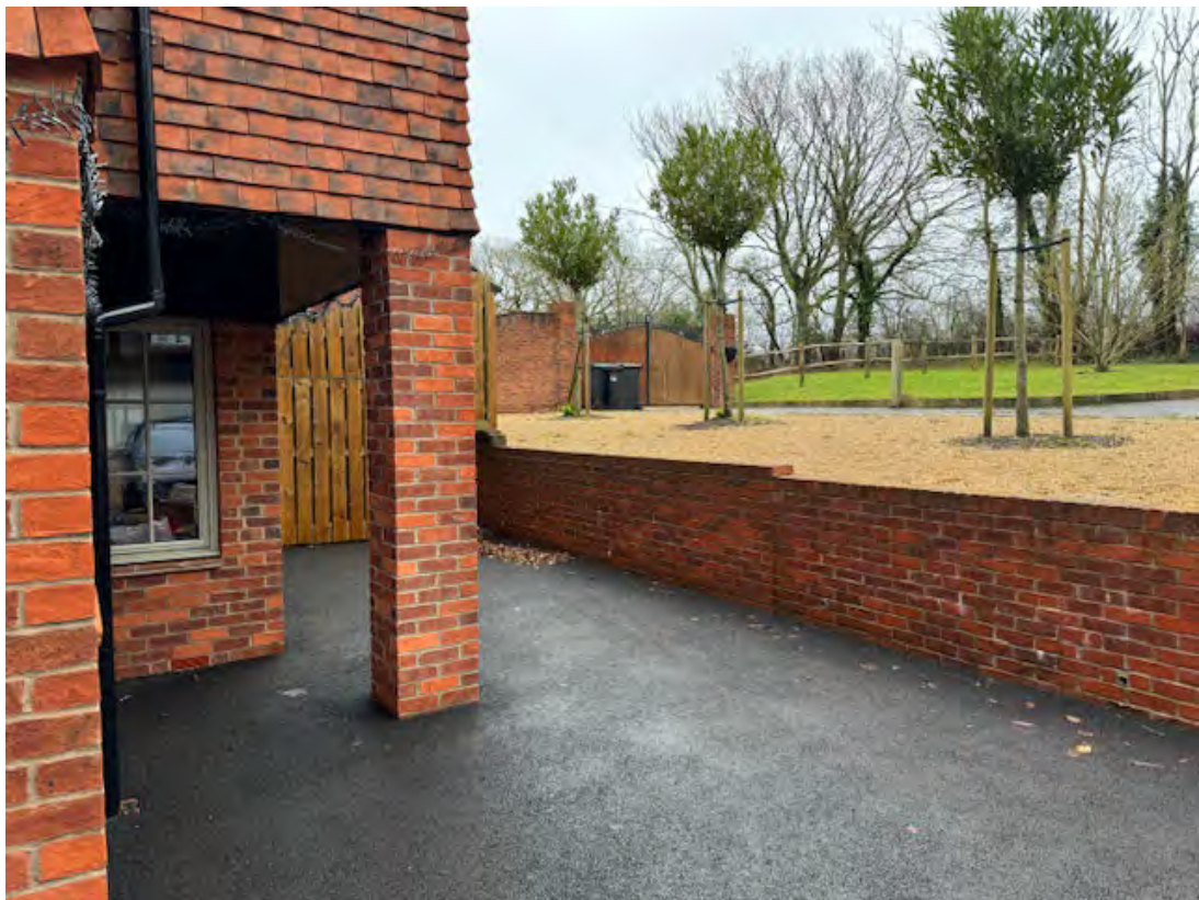
Southern part of site at dwelling entrance
