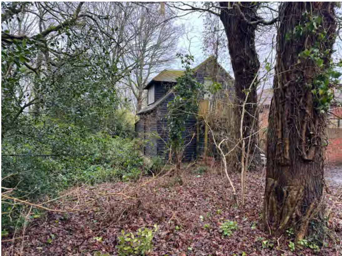
Double garage located in southwest corner of the site
