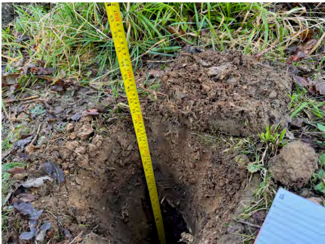
TP2 depth upon completion
