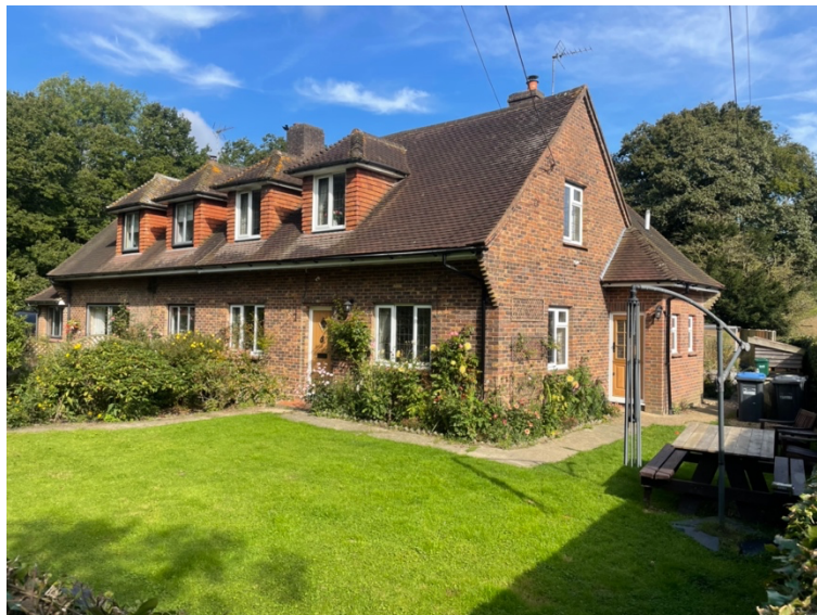
View looking north-west showing front & side elevation
