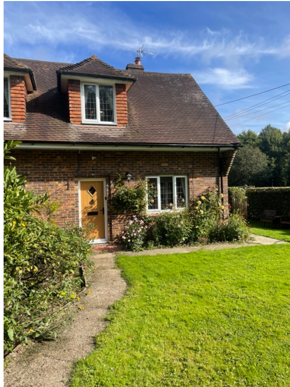
View looking north showing front elevation
