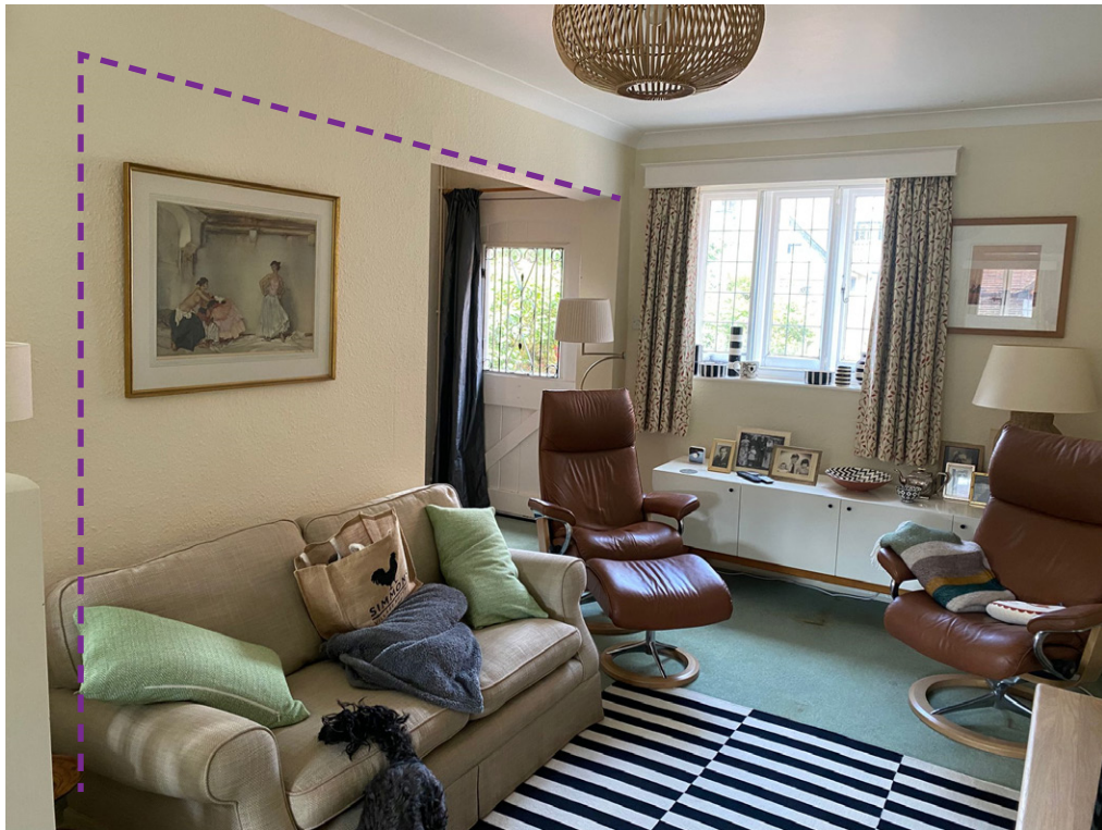
View across lounge towards side entrance door. Proposed extent of opening shown with dotted purple line.
