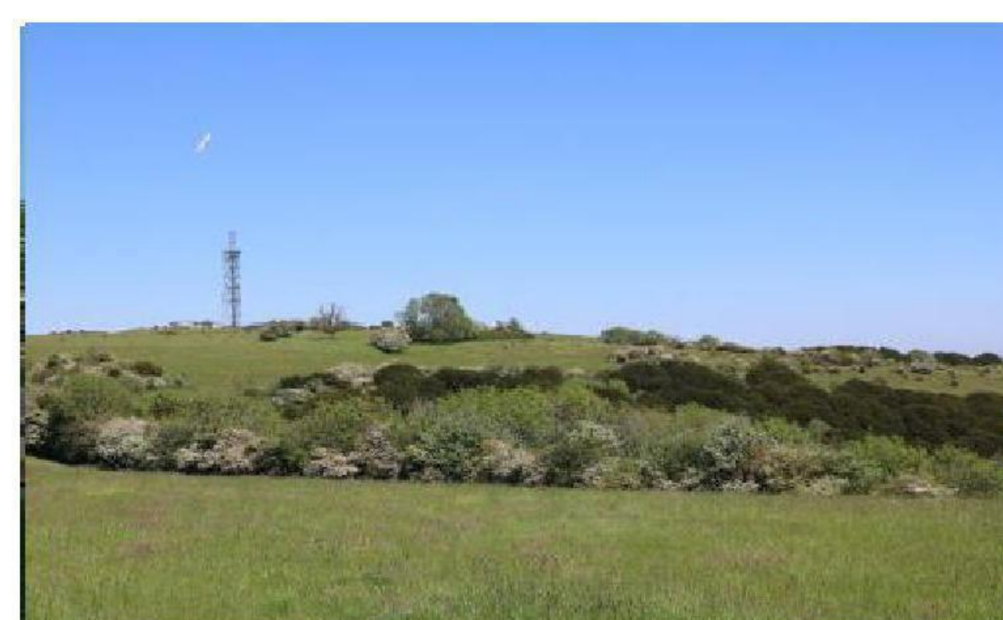
South Downs National Park 10 number Telecommunications Masts
