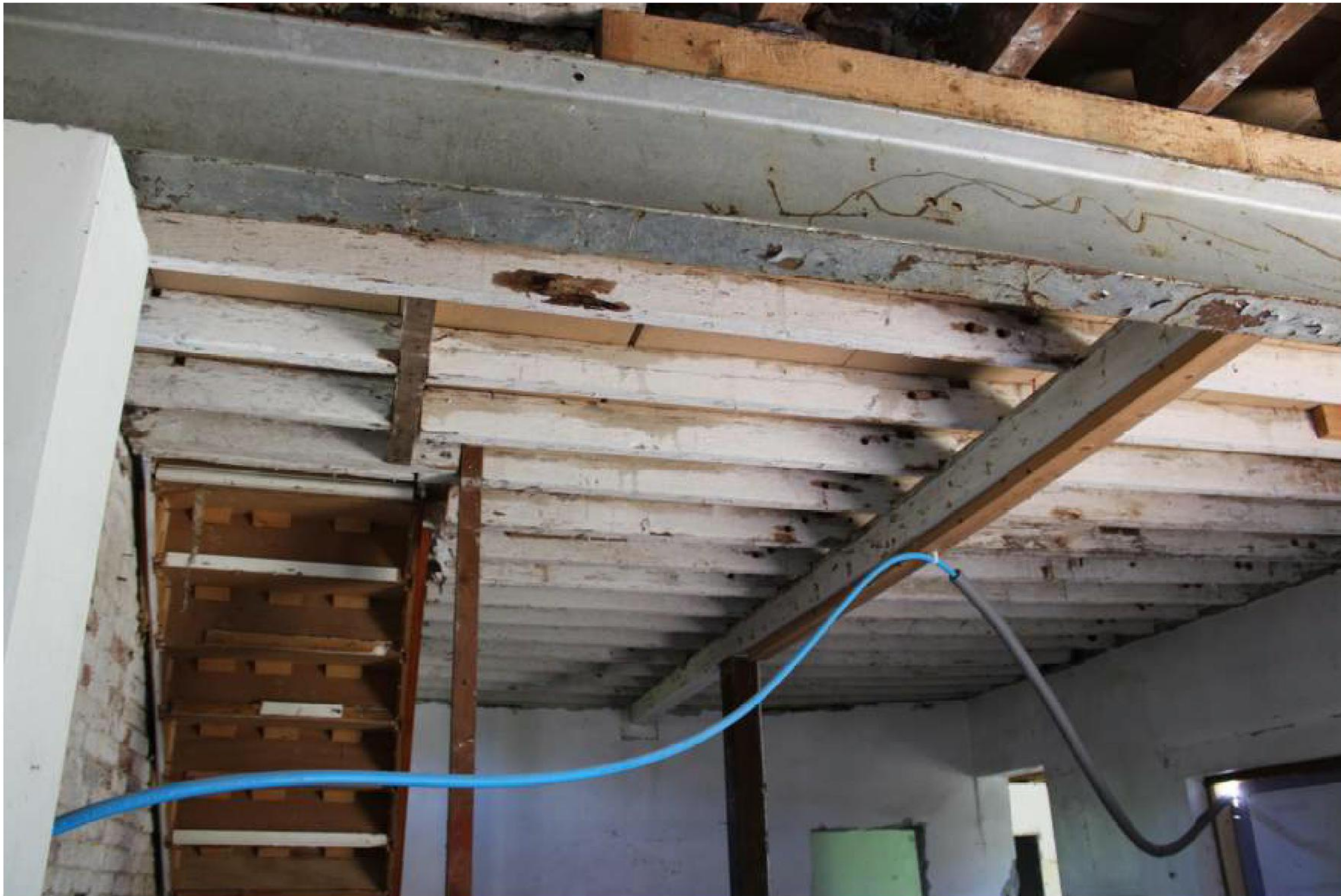
Figure 3 Existing Steel Beam supporting brick wall above and timber beam, which is also supported off the timber column.
