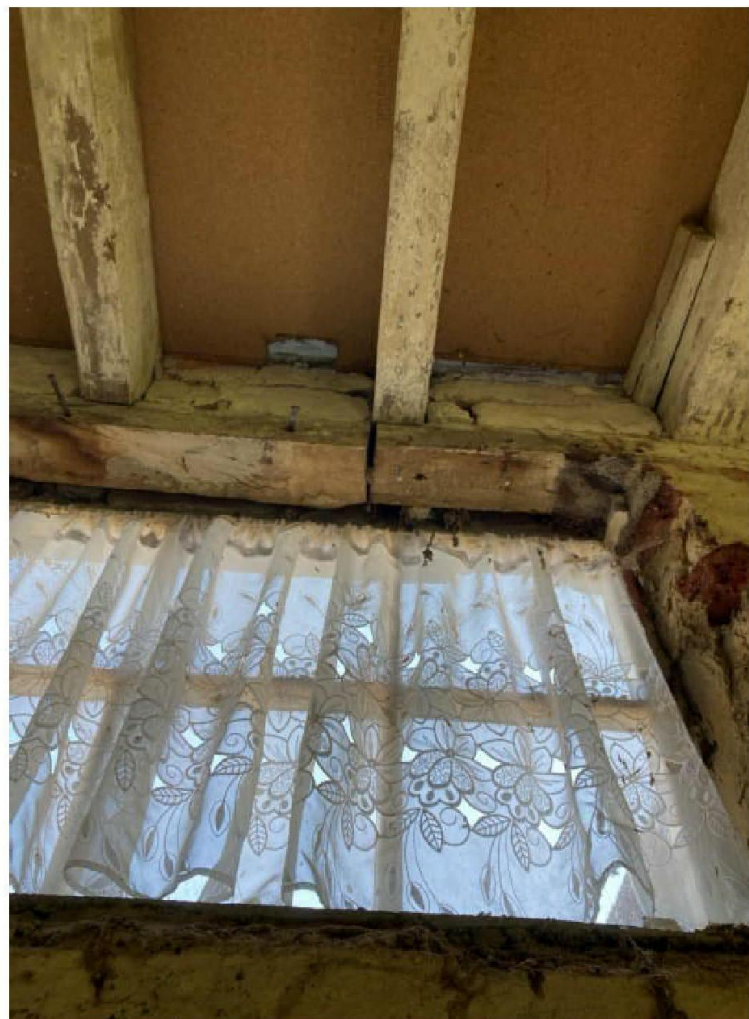
Figure 6 Splice in timber lintel.
