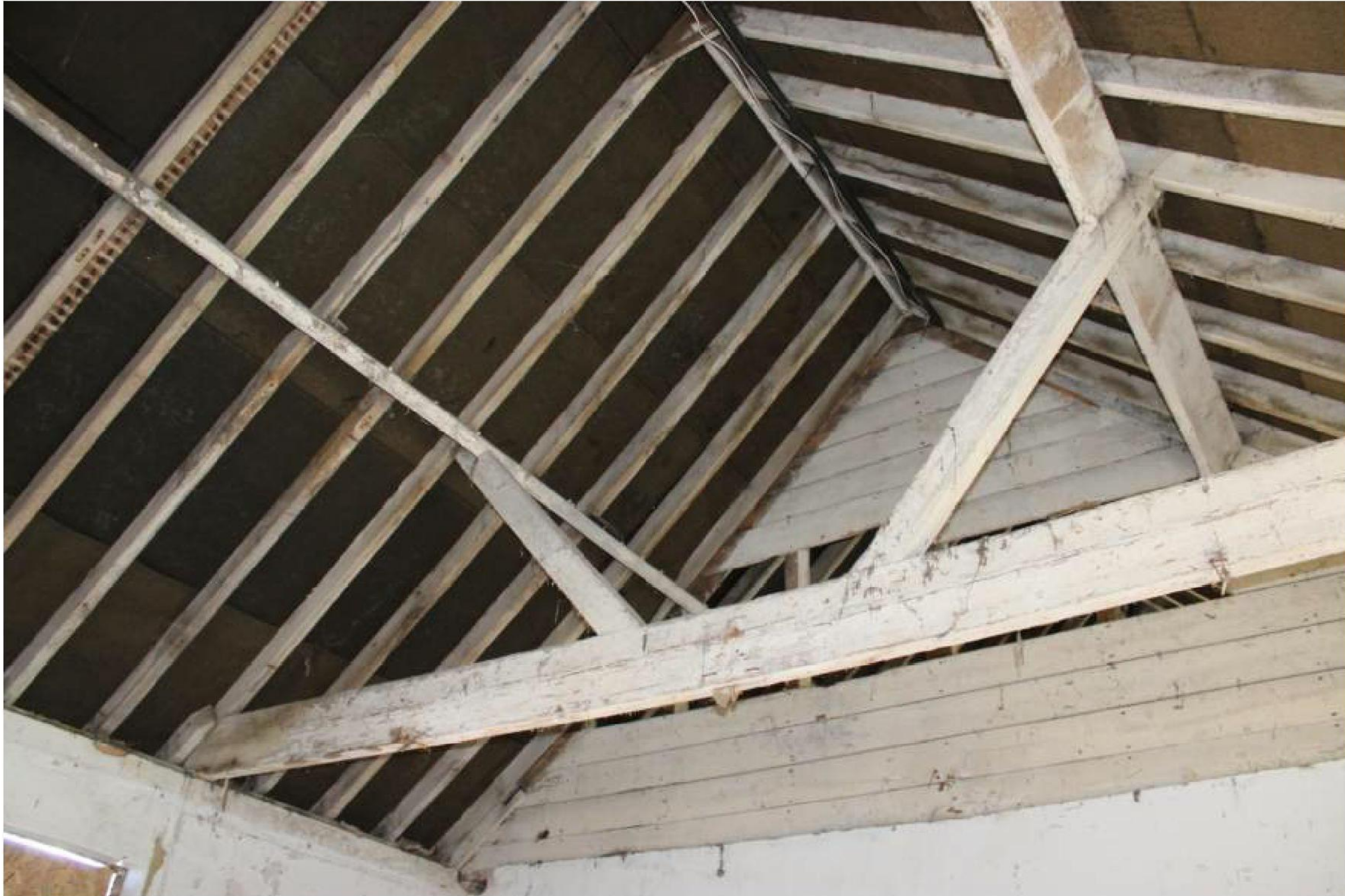
Figure 13 Truss 4 in South Range East.
