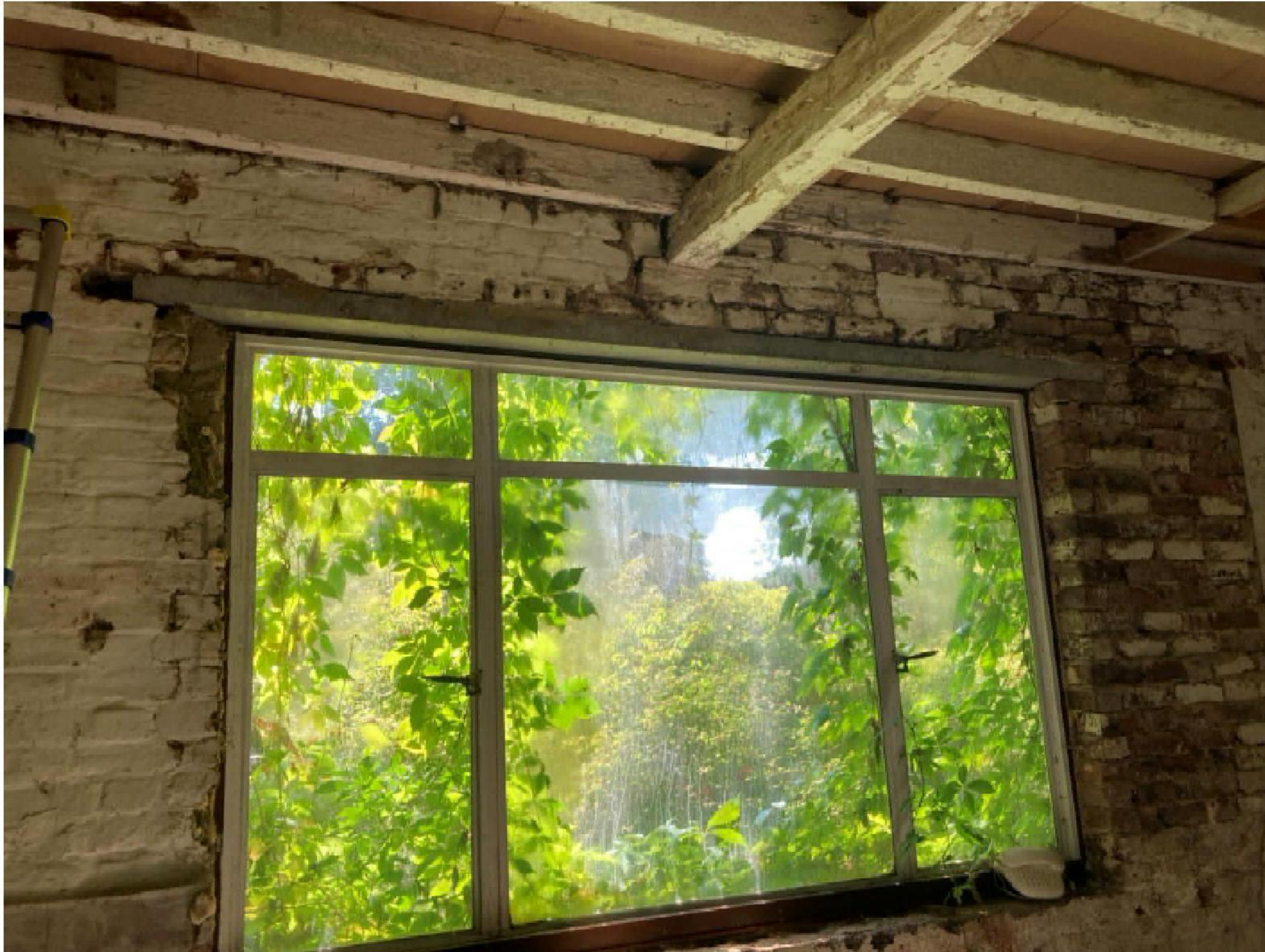
Figure 7 Concrete lintel in the East Range.
