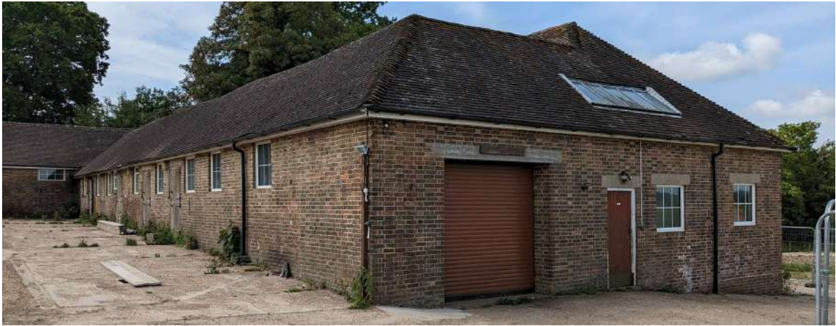
Fig13. View of the north end of the West Range and Barn Store looking southwest
