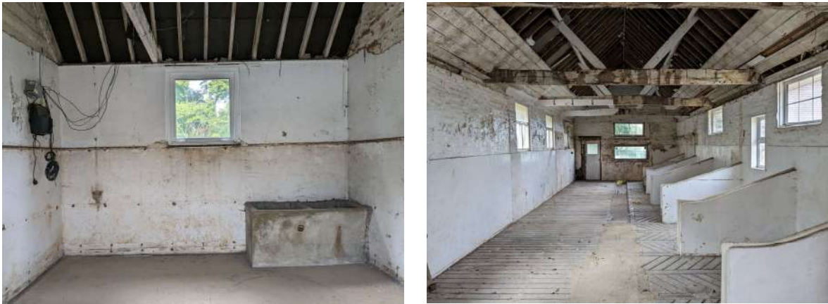
Fig10 & 11. Internal view of the upper and lower stable buildings
