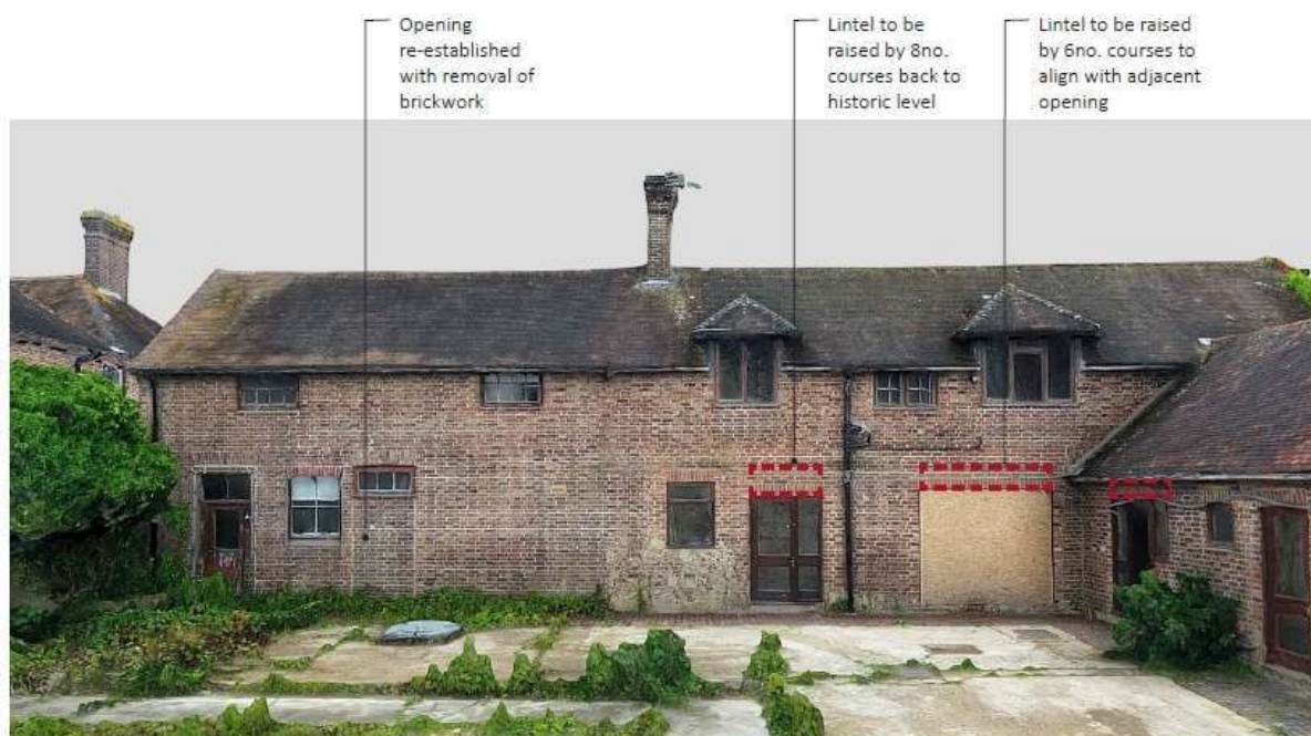
Fig27. View of the lintels to be raised in East Range to align with historic level
