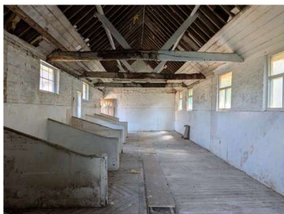
Fig20 & 21. Internal views of the lower South Range showing existing trusses to be retained with stall dividers needing to be removed, looking east & west
