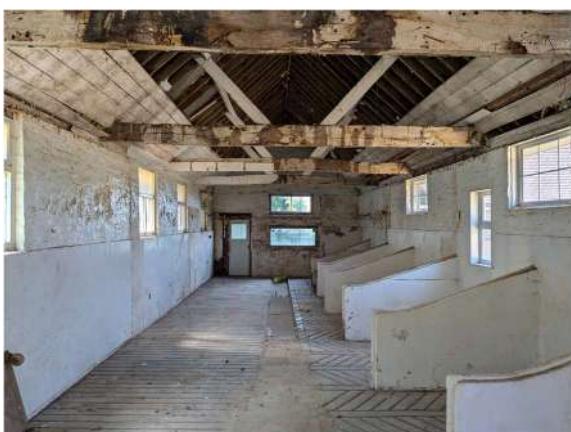
Fig20 & 21. Internal views of the lower South Range showing existing trusses to be retained with stall dividers needing to be removed, looking east & west
