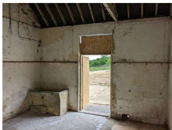
Fig18 & 19. Internal views of the upper South Range showing the trough being retained and the other removed
