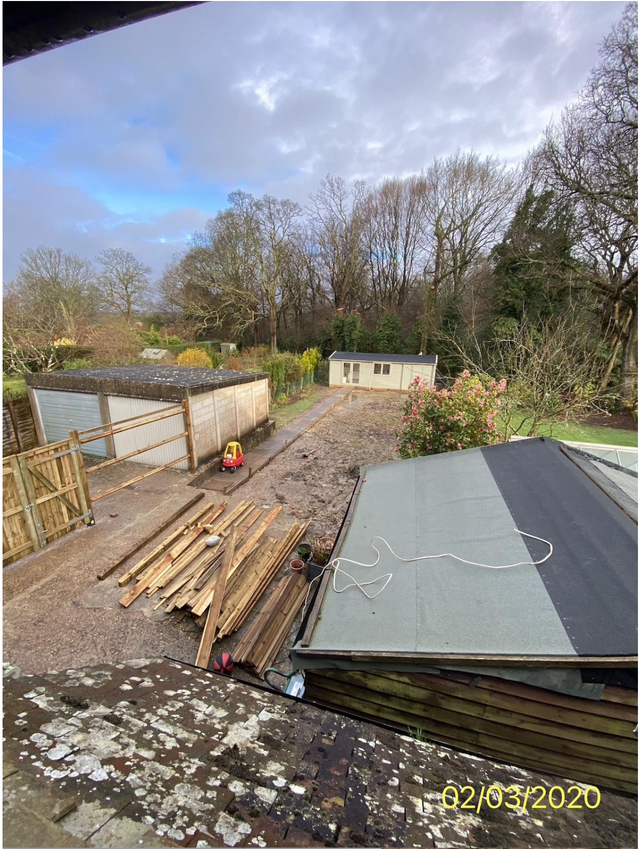
IMG_4276.jpg: External image showing the log cabin in relation to the overall site and that it was complete by 02/03/20.
