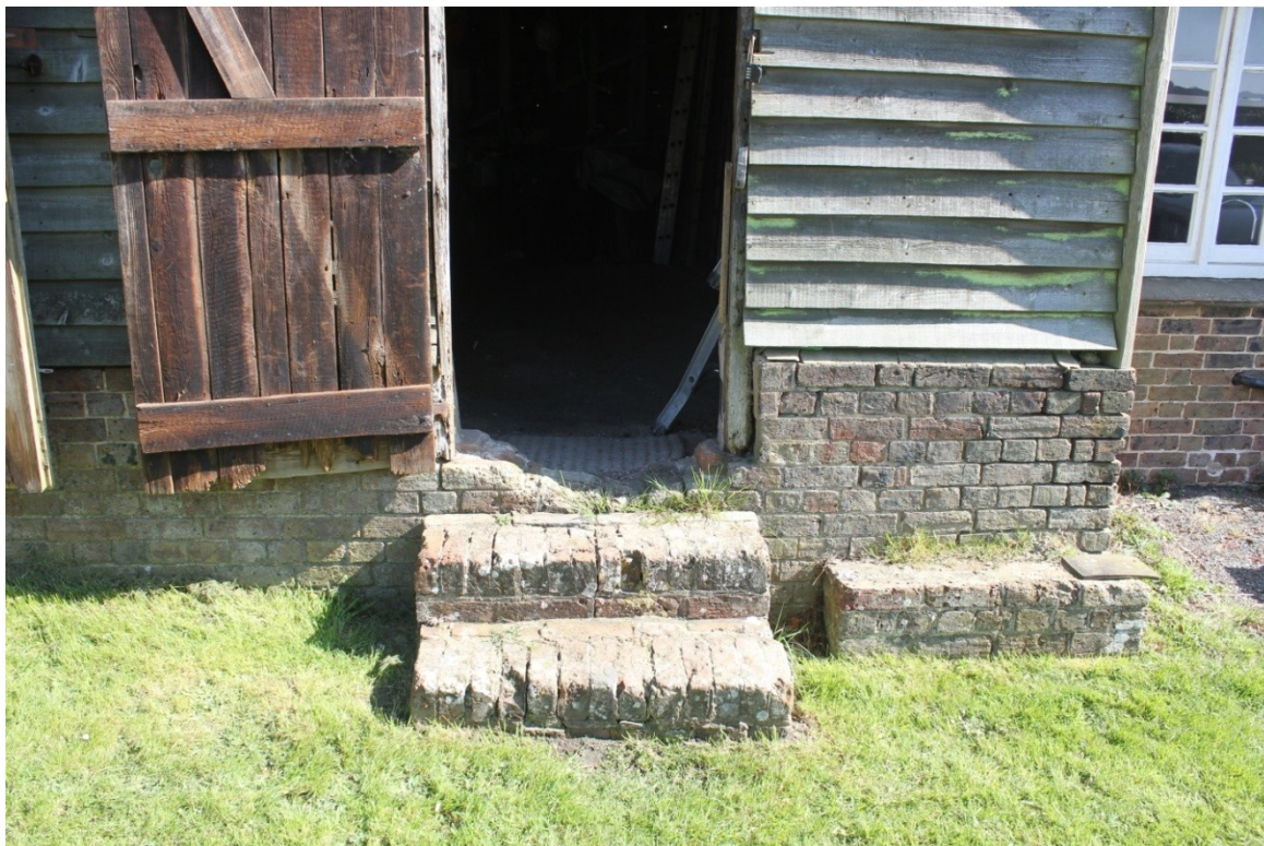
Plate 33. Under-built brick plinth in the west side of the Barn.
