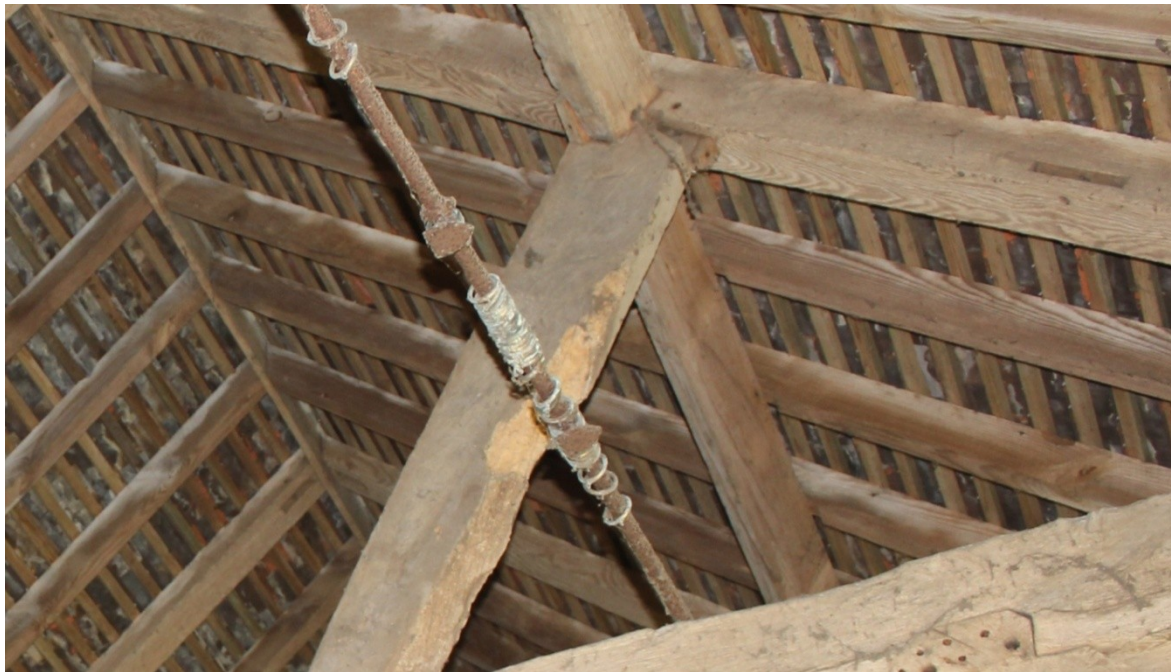
Plate 44. Queen post turned and re-cut with a wedge inserted.
