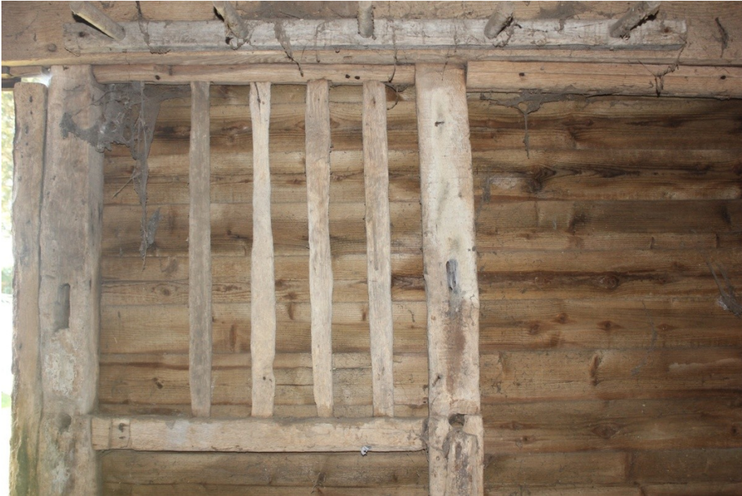
Plate 38. Makeshift mullion window north of the pedestrian doorway to the west.
