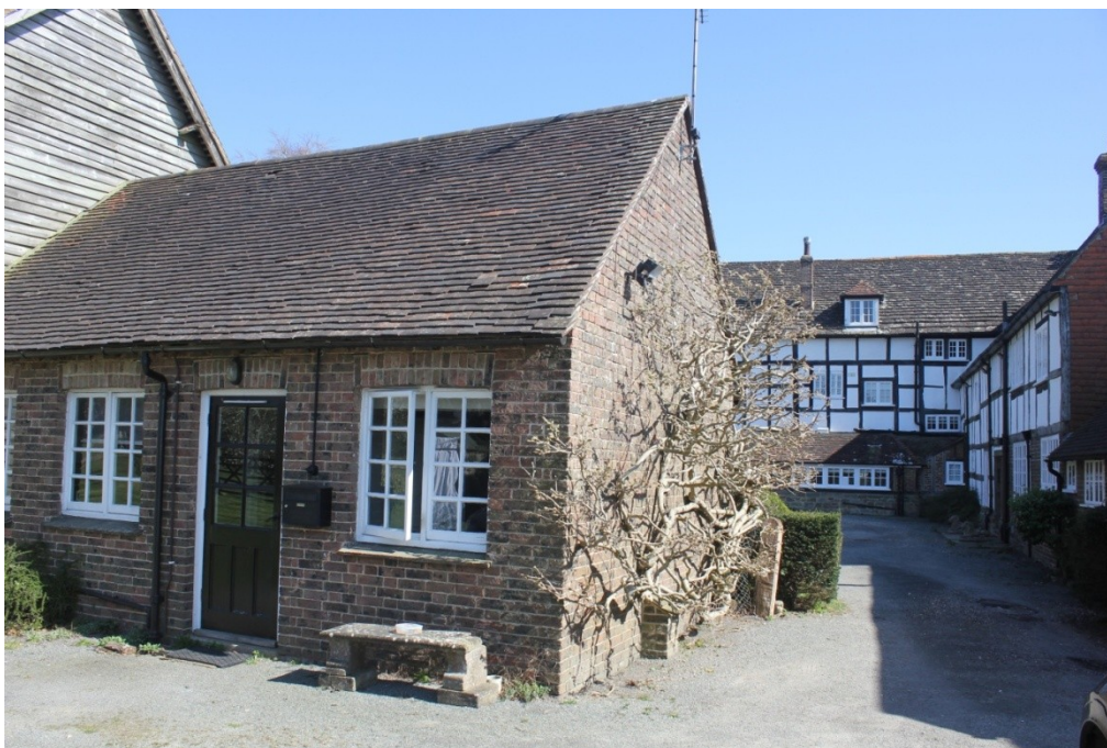
Plate 61. The western elevation of the southern outbuilding.
