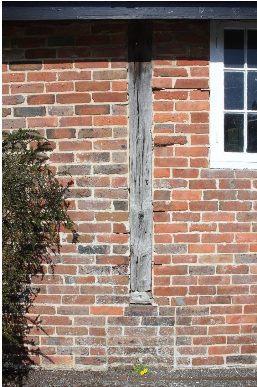
Plate 49. Bay post pad replaced by brickwork at a different date to the infill.
