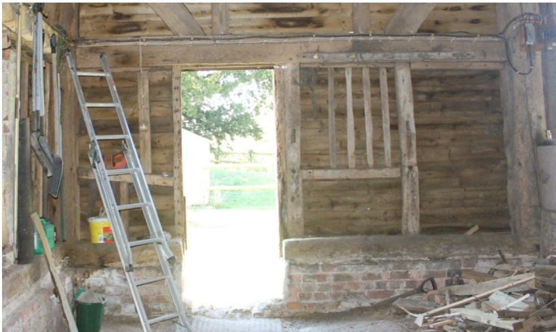
Plate 40. Inserted Period B doorway adjacent to the inserted windows.
