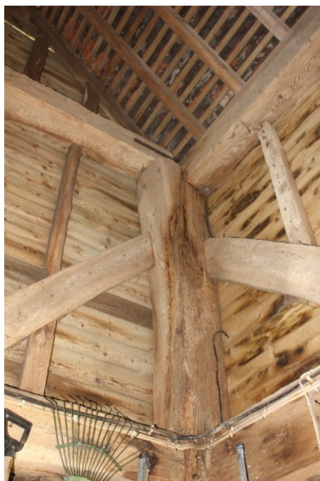
Plate 16. Post A with slightly curved foot bracing.
