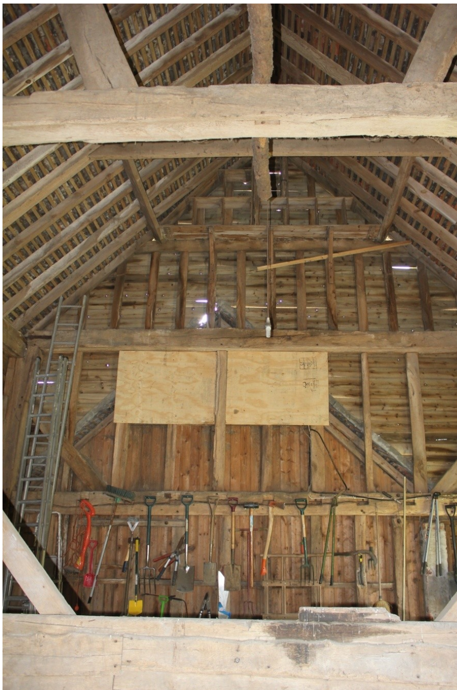
Plate 46. Softwood purlins in the southern bay.
