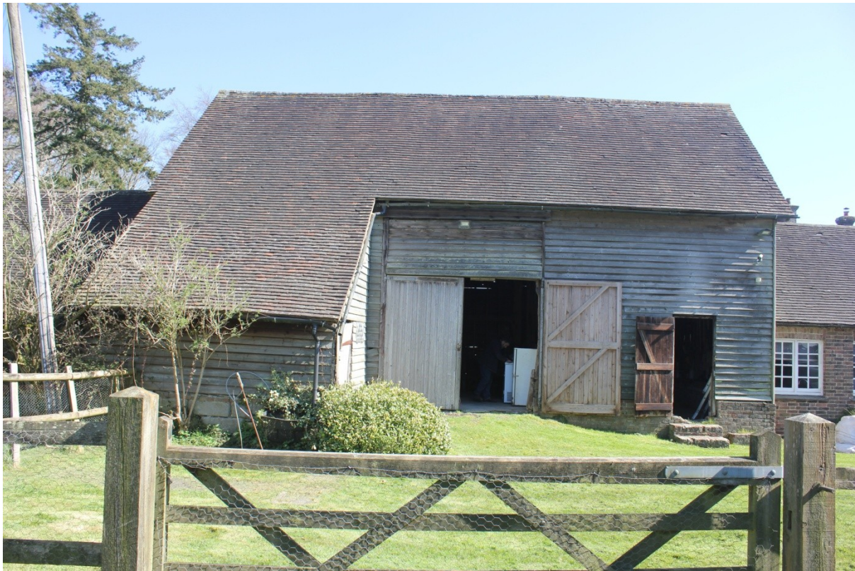
Plate 2. The rear, west elevation.
