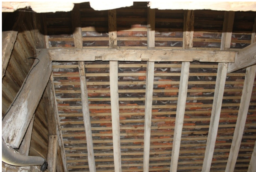
Plate 28. Empty notches from a former wallplate in the outshot purlin.
