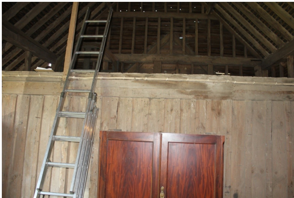
Plate 56. Period C plank and muntin wooden partition wall in Truss C.
