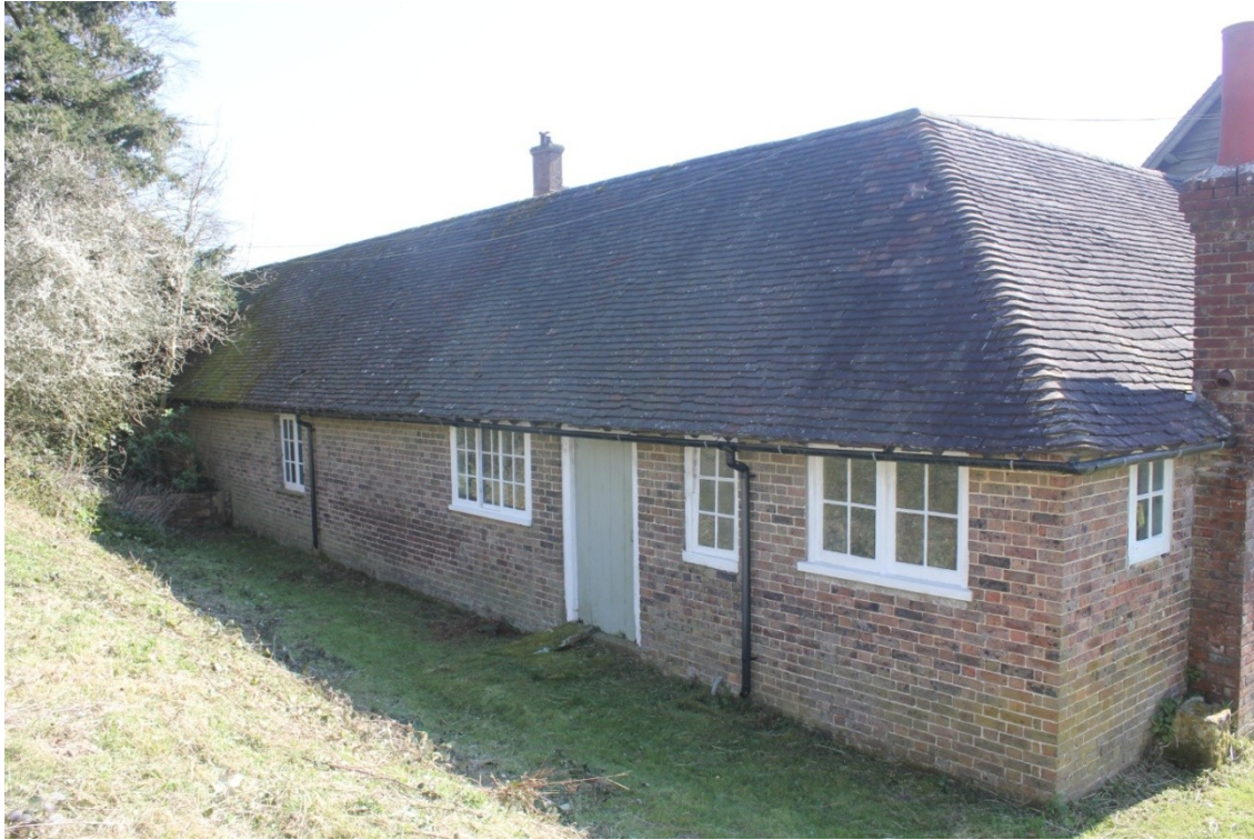
Plate 52. Windows and doorway in the northern elevation.
