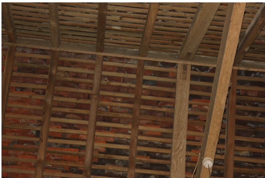
Plate 42. High set collar mortices at the ridge.
