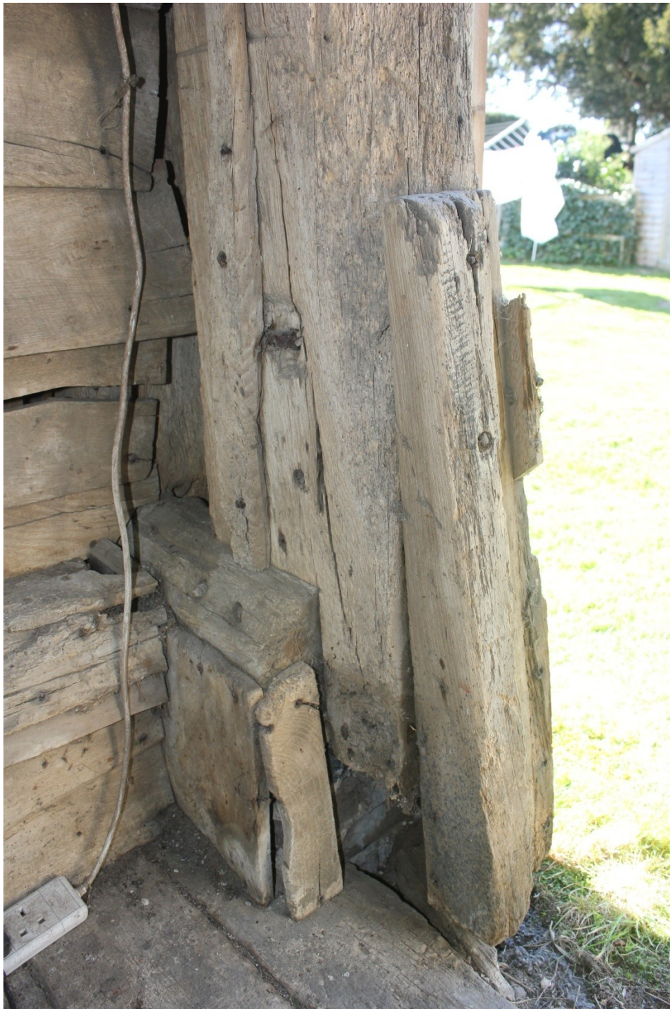
Plate 20. Southern 'slide' in-situ on Post B.
