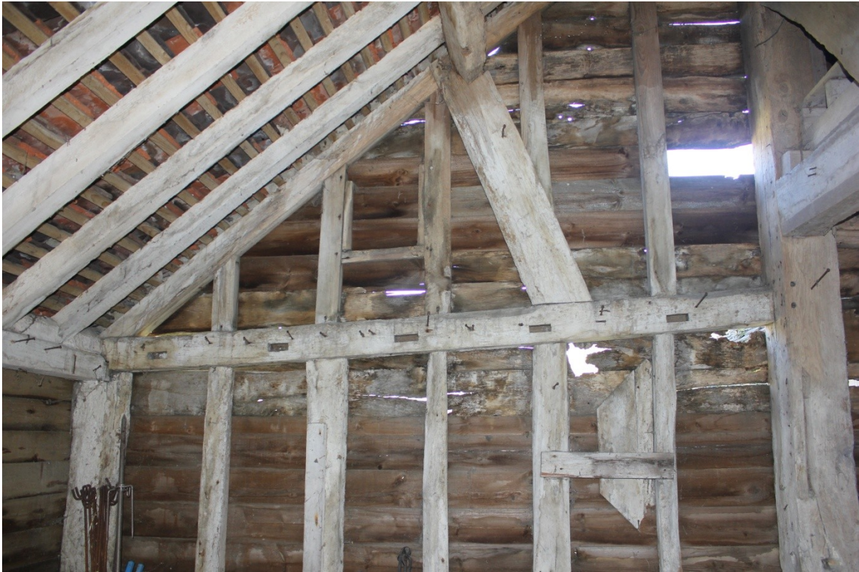
Plate 27. Joist mortices in the northern tie.
