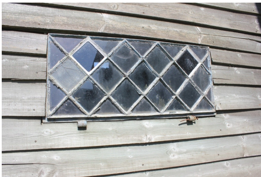
Plate 32. Re-used, inserted window in the outshot southern wall.
