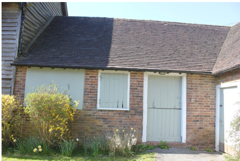
Plate 8. Outbuilding to the north.
