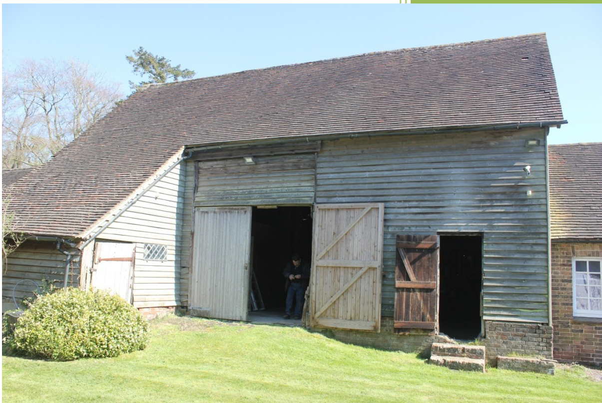
The rear, west facing elevation.
