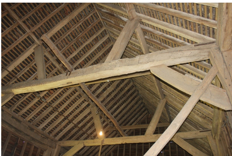
Plate 23. The level roof structure with Truss B in the foreground looking towards Truss C.
