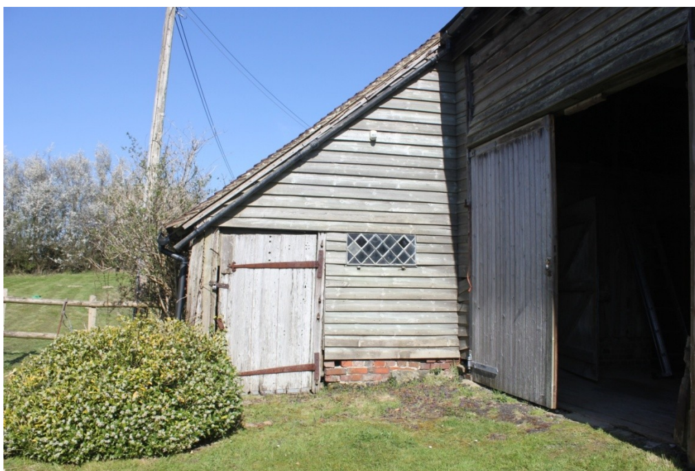
Plate 30. The southern wall of the Outshot.
