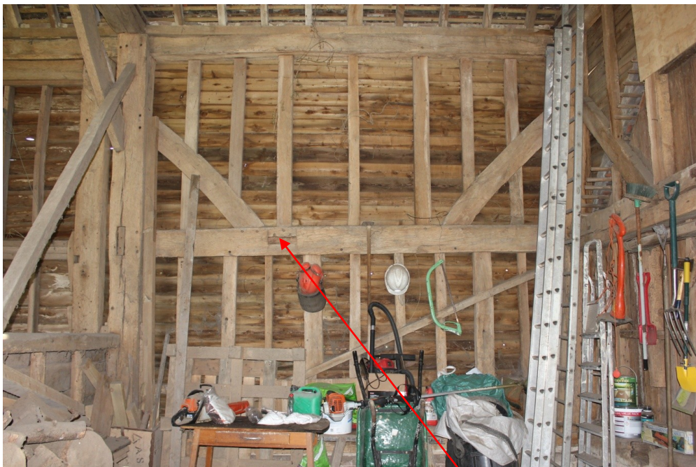
Plate 13. The east wall of the south bay with empty mortice for the floor plate.
