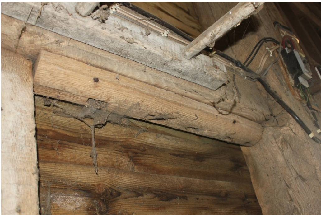
Plate 39. Re-used ovolo moulding in the second window head.
