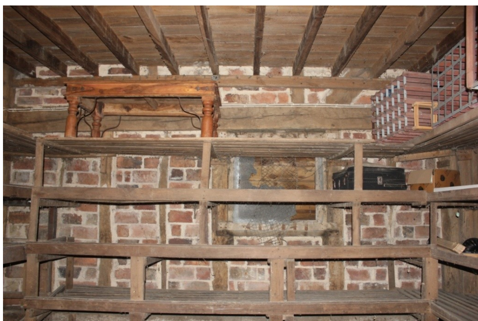
Plate 57. Window inserted in the eastern wall.
