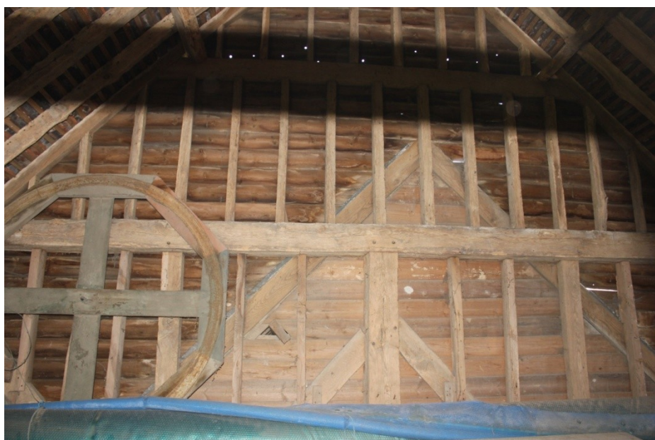
Plate 43. The northern outbuilding built against the gable.
