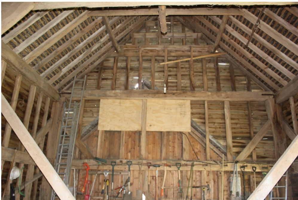
Plate 11. The southern wall of the South Bay.
