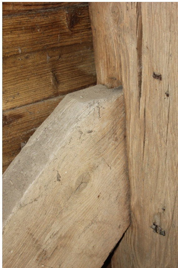
Plate 3. Curved brace with shoulder at the mortice and tenon joint.
