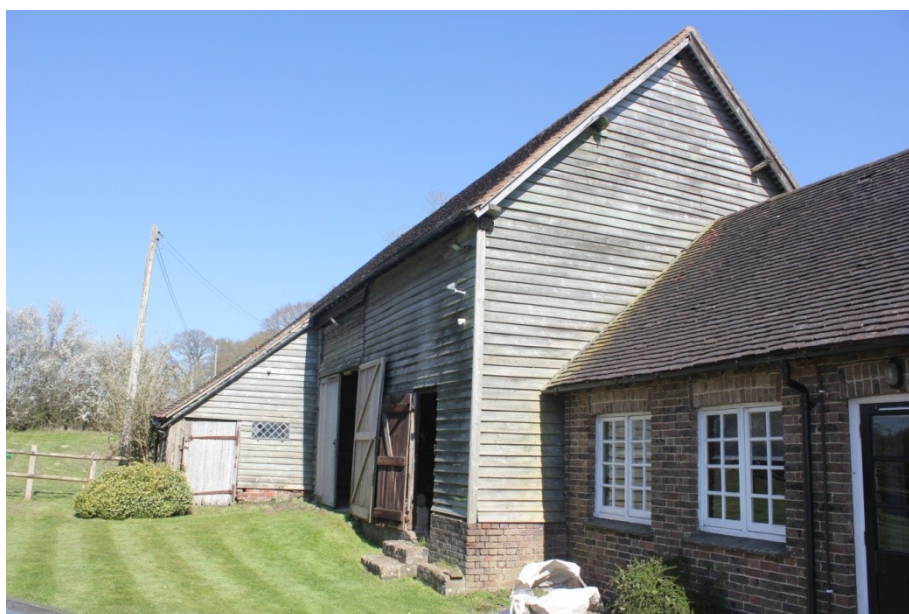
Plate 4. Early 20 th century outbuilding attached to the south elevation.
