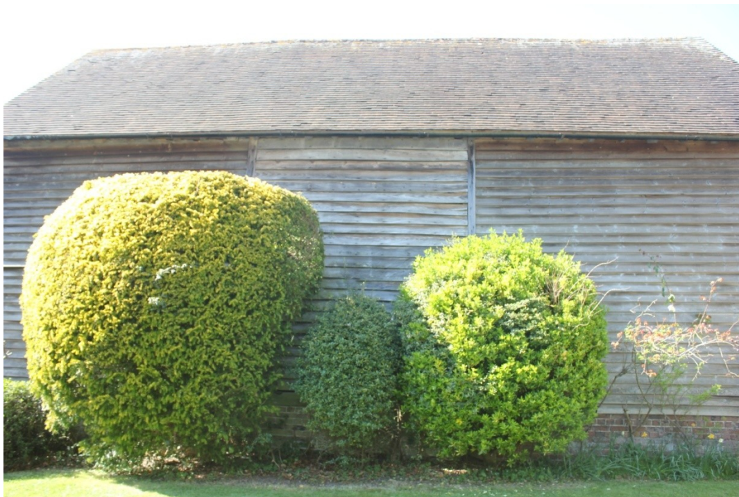
Plate 6. Infilled Midstray to the east.
