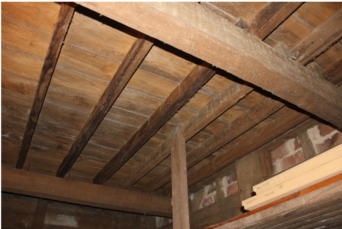
Plate 58. Period C floor inserted into the northern bay.
