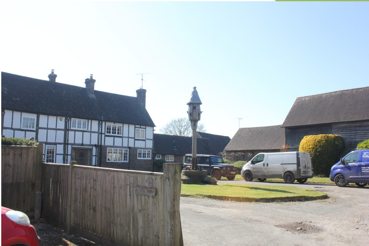
'Keysford' next to the Barn situated within the former farmyard with the Barn on the right.
