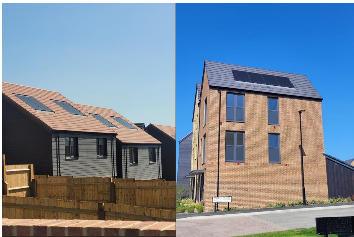
Figure 2: PV Examples on Vistry Development, Burgess Hill
