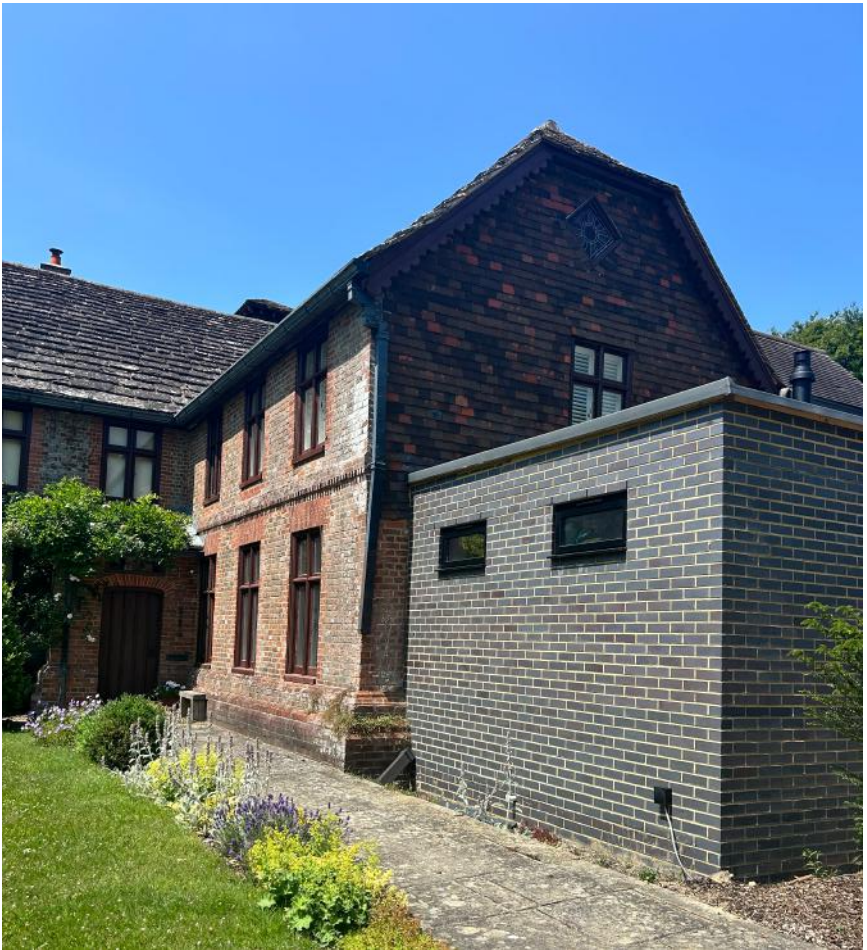
As currently built South Elevation N.B. project still under construction, yet to be completed.
