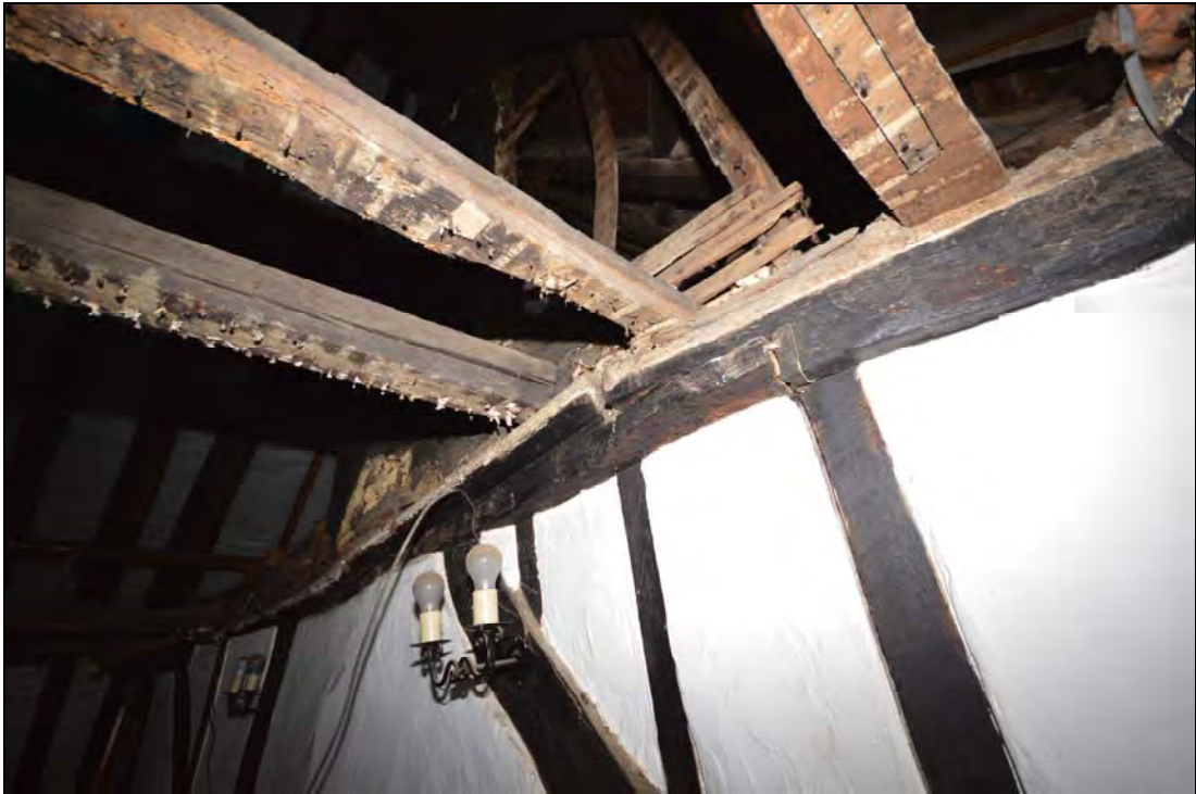
Plate 25: Detail of the bearer attached to the wall plate/tie-beam of the T2 truss/southwest wall plate between the main range and cross-wing
