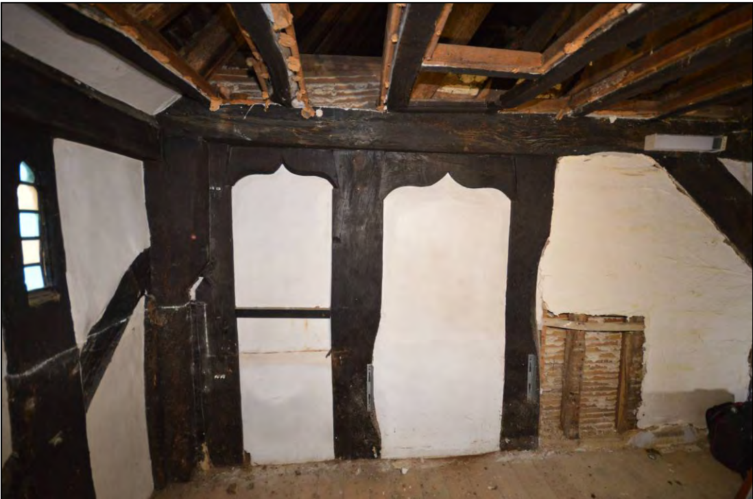
Plate 11: The two adjacent doorways at first floor level in the T5 truss viewed from within the northwest end bay (bay 5; Figure 8)
