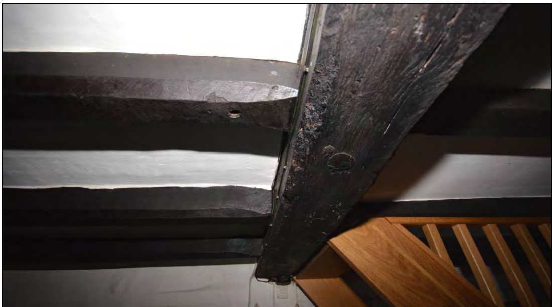
Plate 20: Detail of the surviving joists of the first floor structure in bay 6
