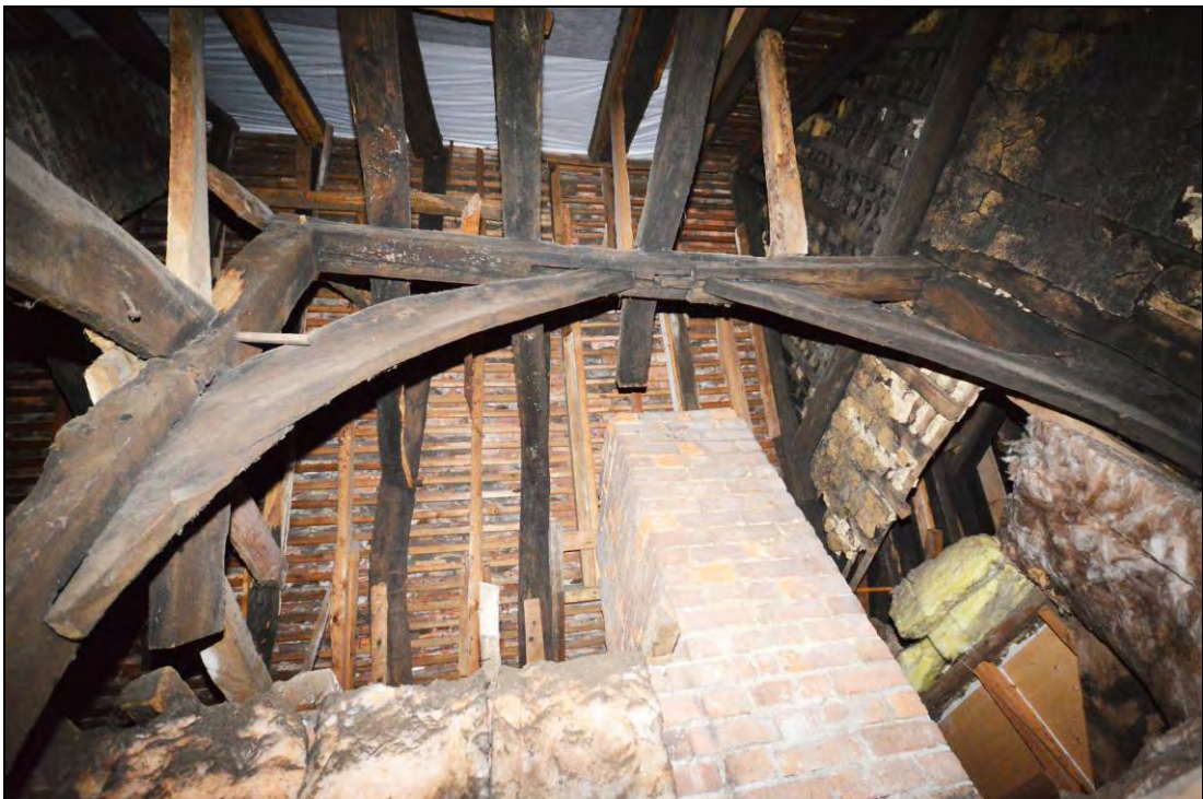
Plate 16: The roof over bay 6, the southwest end of the hall rebuilt during phase 2 to create an attached kitchen
