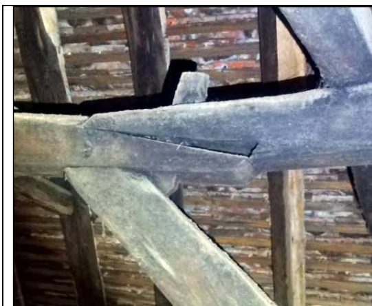
Plate 3: The base-cruck truss (T1) between bays 1 and 2 of the main range (the hall)
