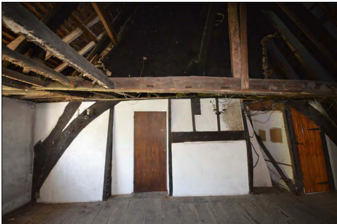
Plate 26: Detail of the girder spanning the width of bay 2 from the inserted flying plate to the southeast to one of the rafters in the northwest roof slope; also shows two of the suspending members used to support the girder
