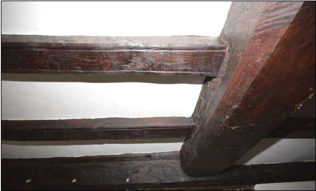
Plate 19: Detail of the inserted floor added to bay 1 of the hall to create a chamber above, note the moulded detail to the robust joists.
