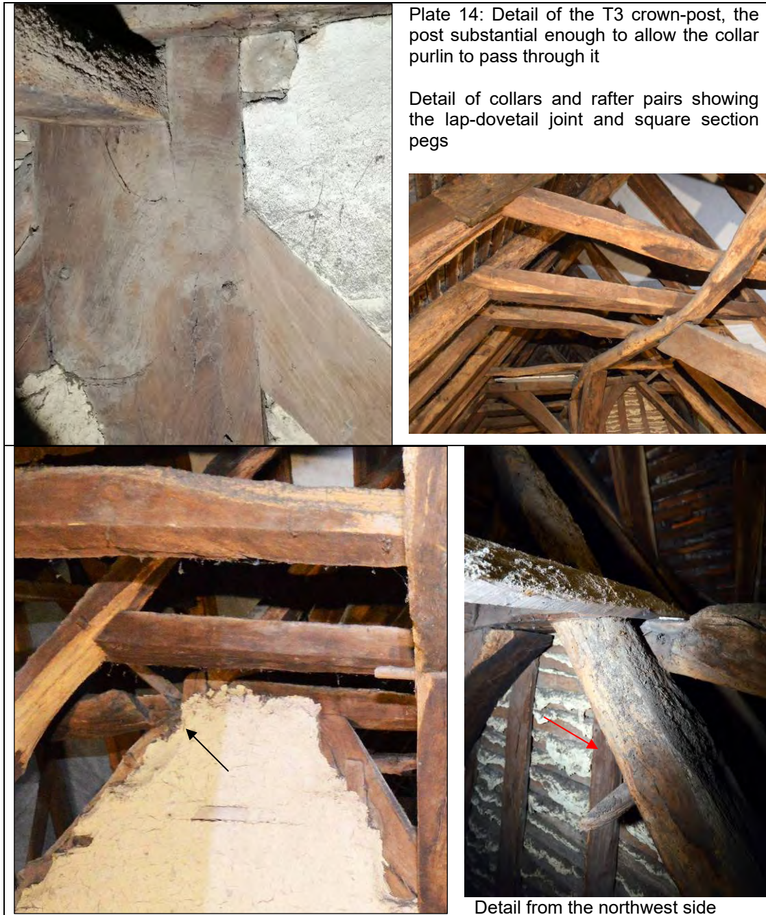
Plate 15: The tenon with its central peg-hole situated at the end of the collar purlin at its junction with the former open truss (T4) of the cross-wing (black arrow). The detail shows the same junction from the northwest side of the truss, in addition to a robust peg that had been driven through the rafter below the junction of the two roof structures (red arrow)
