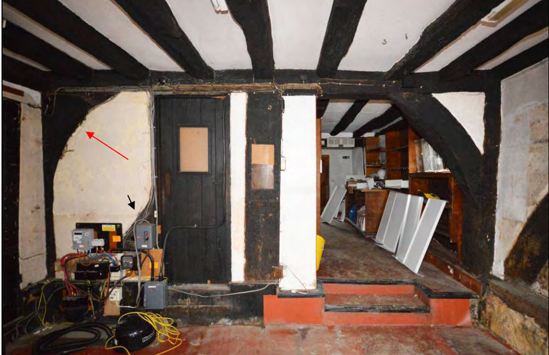
Plate 10: The T4 truss on the ground floor showing the central stud, braces, and durn-type bracket (red arrow), the surviving base of the foot-brace just visible behind the meter (black arrow)
