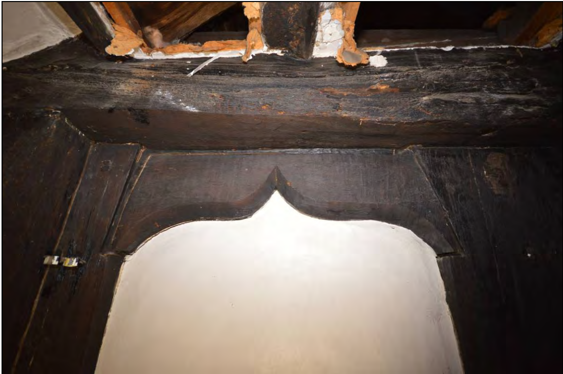
Plate 12: Detail of the chamfered leading edges of the ogee door-heads and the squinted abutments to their jambs (northwest side)
