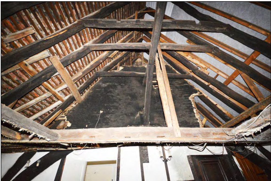
Plate 5: The roof over the hall looking towards the base-cruck truss and the soot-blackened partition inserted in phase 2
