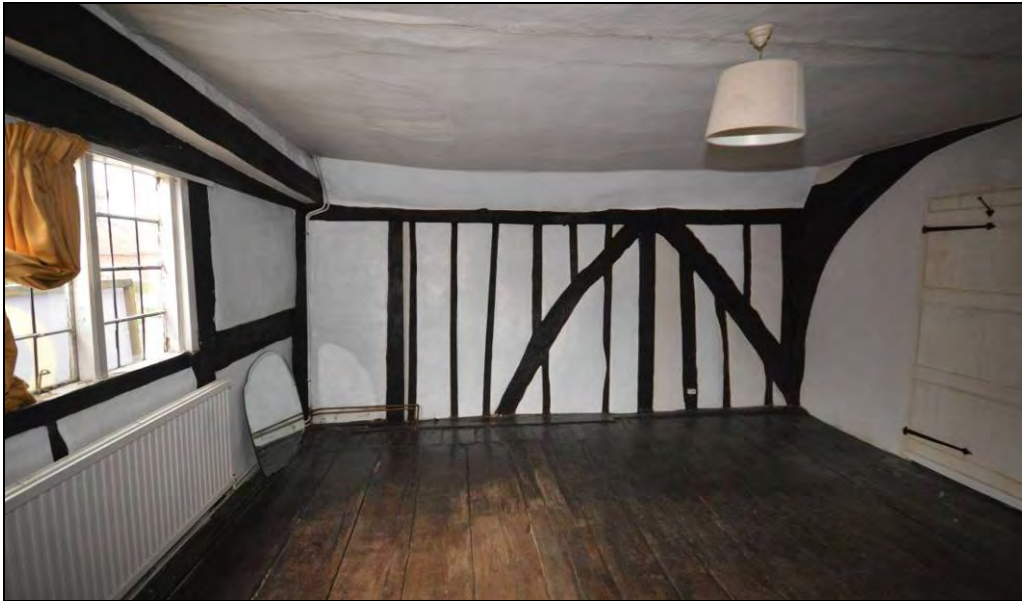
Plate 7: The southwest wall of the cross-wing at first floor level, and an oblique of the street-front elevation and its Georgian window
