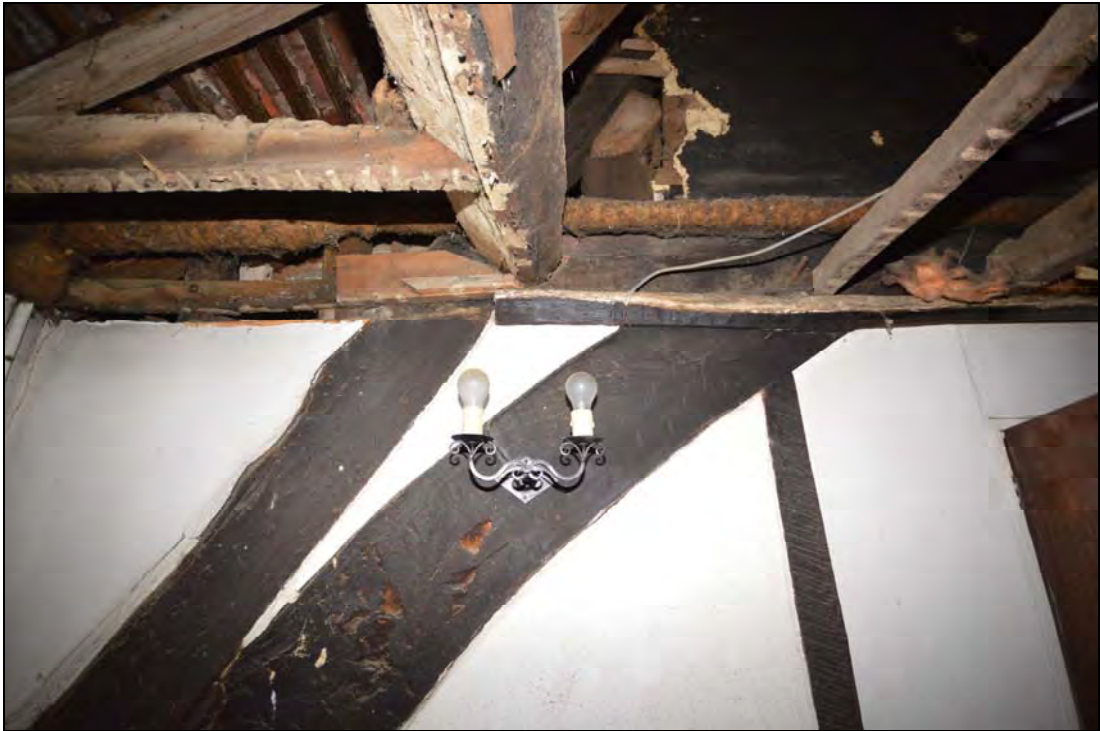
Plate 27: The junction of the inserted flying plate at the southeast side of bay 2 with the 14 th century base cruck truss
