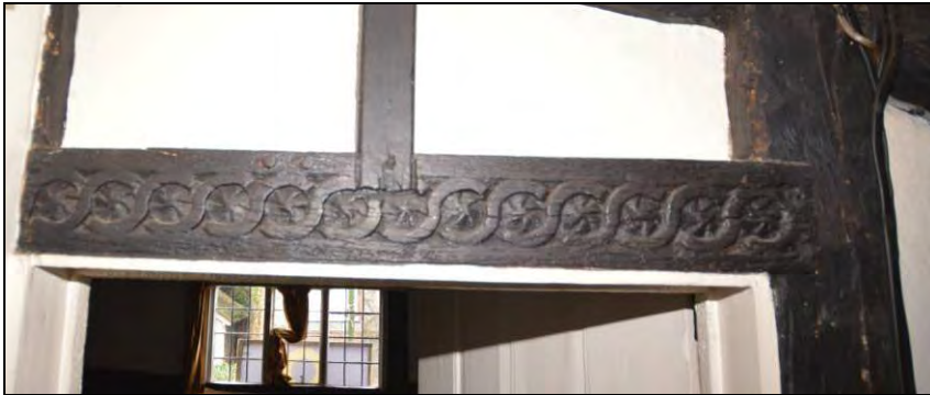
Plate 21: Decorative strap-work over the doorway in the T5 truss
