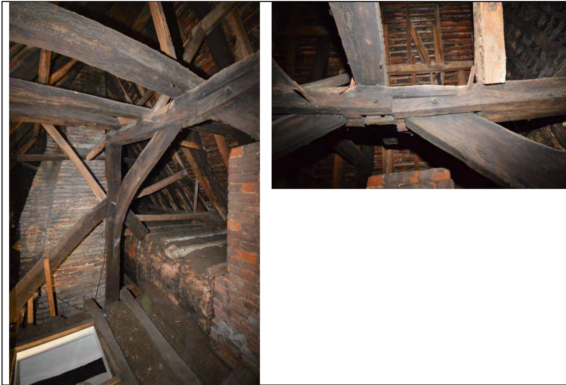
Plate 17: The T7 crown-post and detail of the scarf to the collar purlin between it and T8
