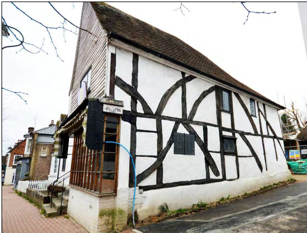
Plate 6: The cross-wing showing the jetty and the wall framing, the jetty under-built to create a shop front
