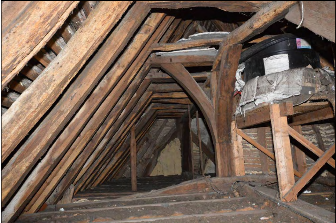
Plate 9: The interior of the cross-wing roof looking to the southeast gable, its substantial crown-post and flanking cross-bracing with the four-way braced truss over the two-bay hall at the centre
