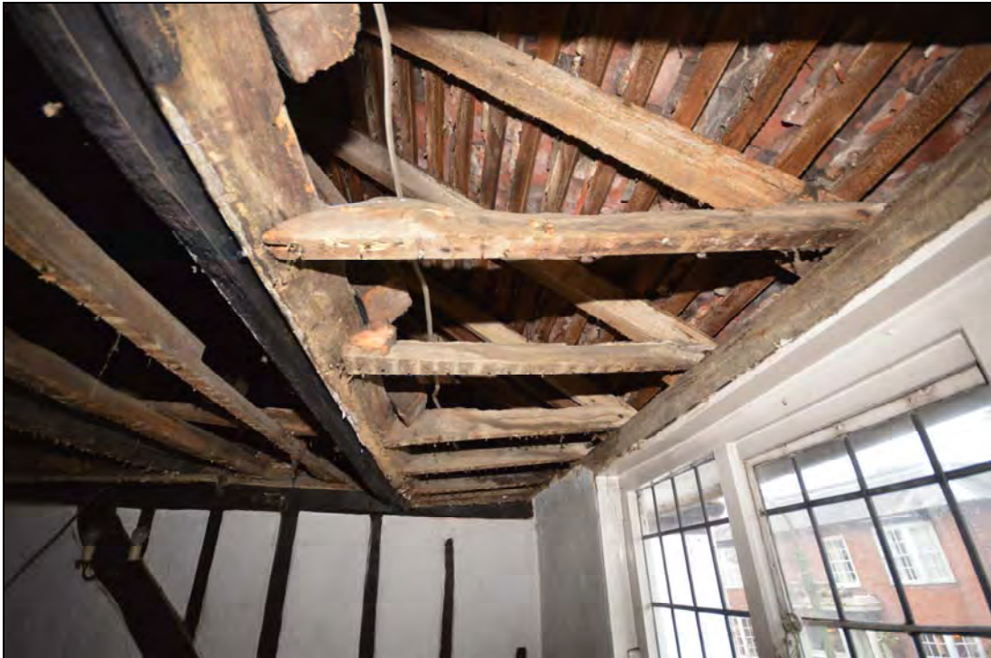
Plate 29: Short lengths of ceiling joists between the inserted southeast plate and the wall plate over the front wall
