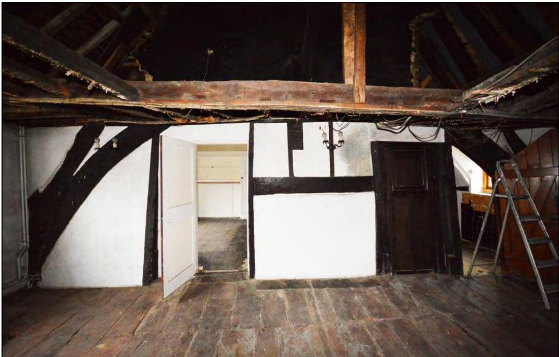
Plate 3: The base-cruck truss (T1) between bays 1 and 2 of the main range (the hall)
