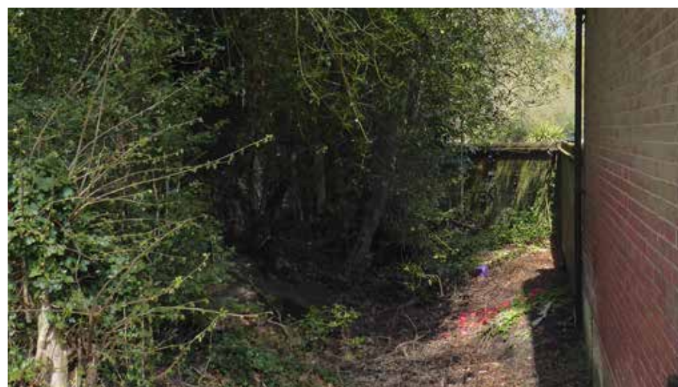
FIG.09 View of the western boundary of Stables Cottage
