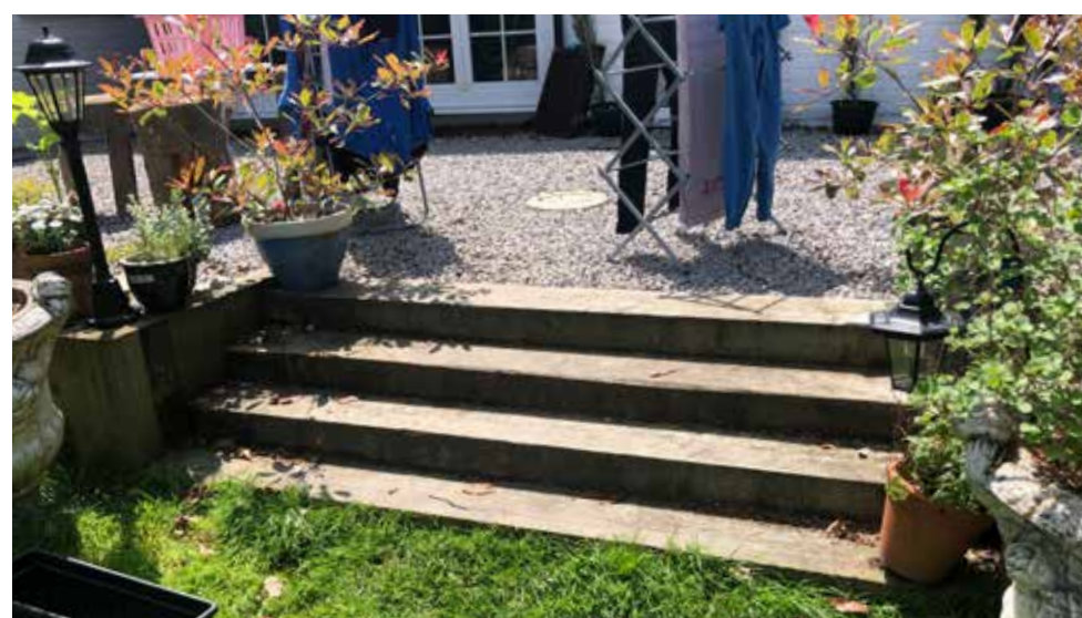
FIG.11 View of steps from garden level up to raised patio area
