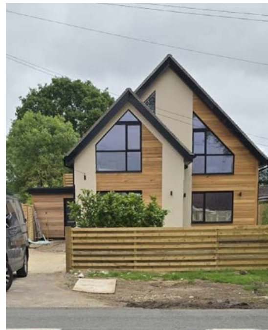
Fig. 18 - 44 Ockley Lane, Hassocks - Approval nearing completion
