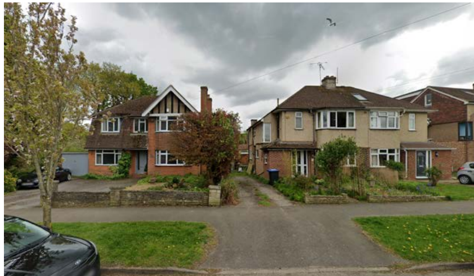
Fig. 7 - Typical properties on Grand Avenue
