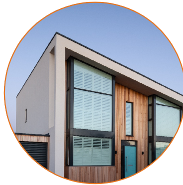
White render surround Aluminium capping + Vertical timber cladding
