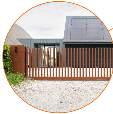
Metal sliding gate + boundary Corten or powder coated steel Colour to match elevation detailing
