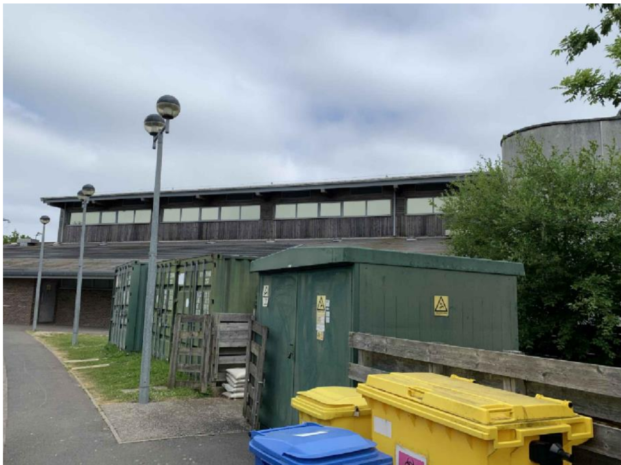
Proposed location, adjacent to plant room and Sub Station
