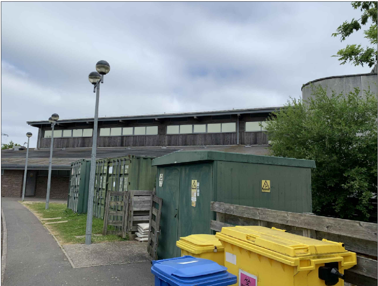
Image to proposed location, adjacent to plant room and Sub Station
