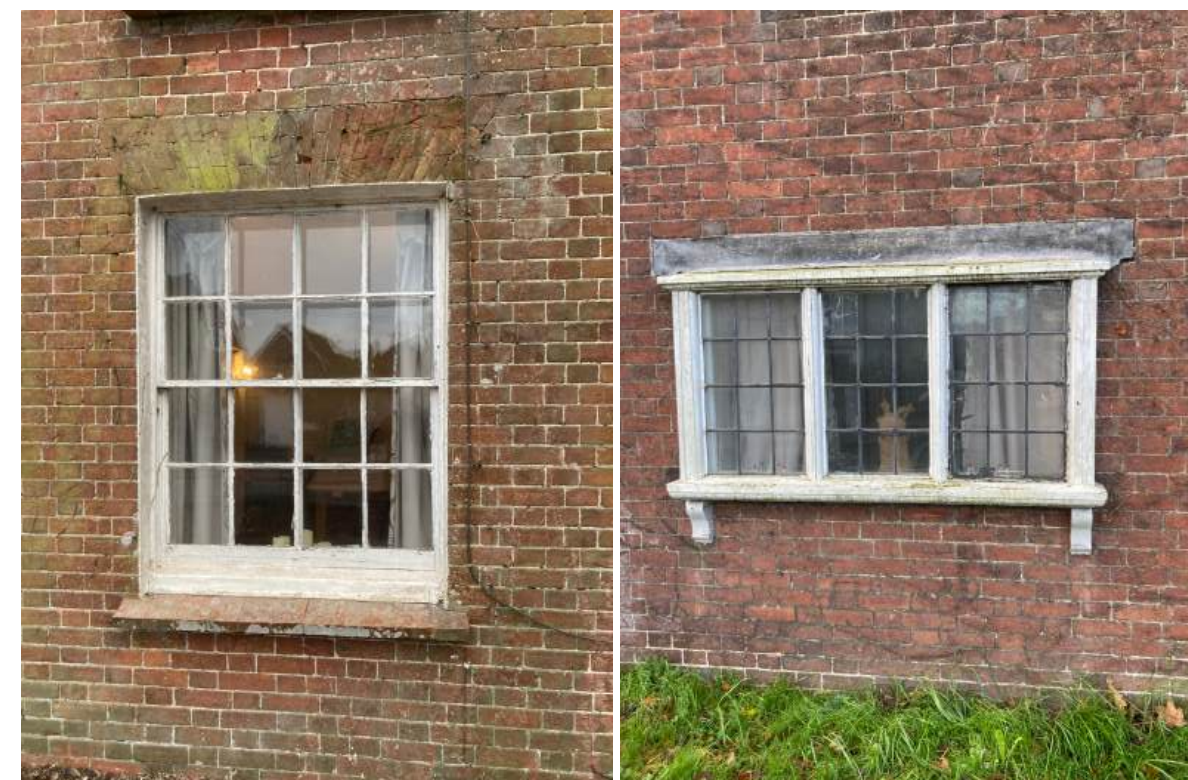
Example of historic windows to be repaired.
