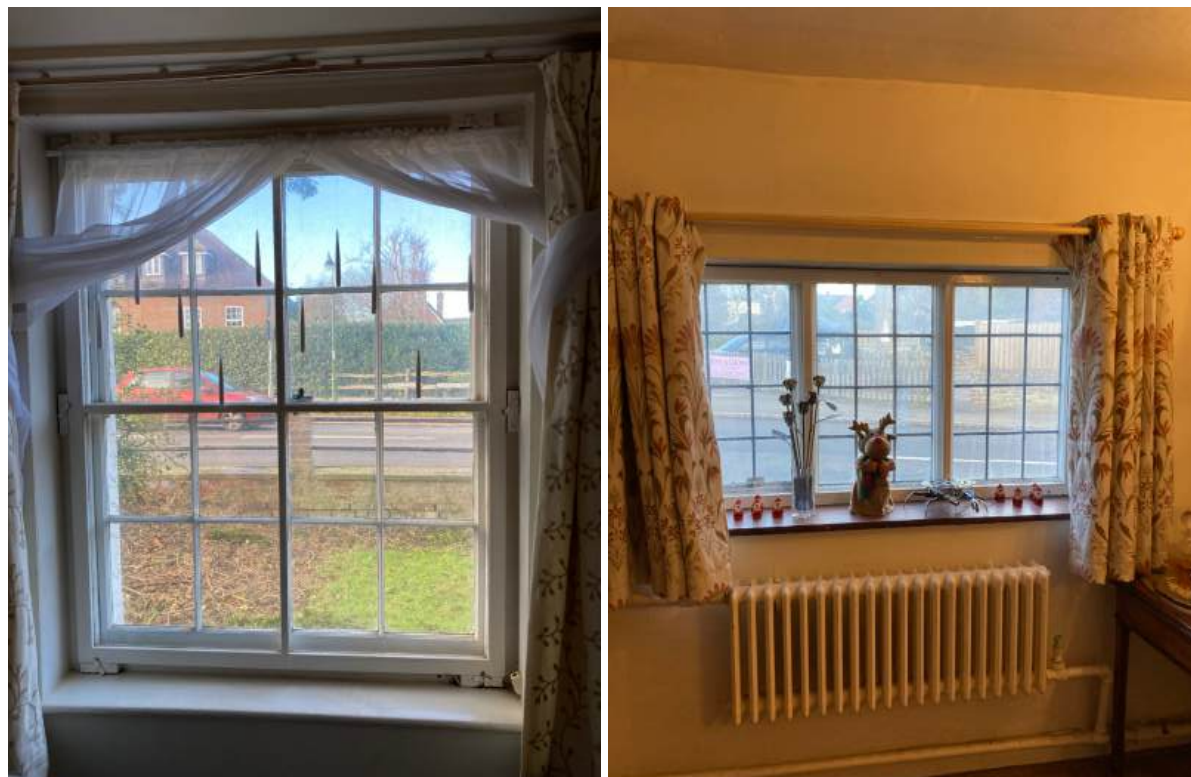
Examples of existing secondary glazing to be replaced.
