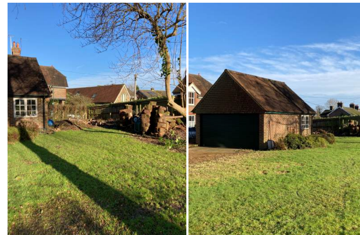
Location of proposed outbuilding (left) and garage building to have photovoltaic panels (right).
