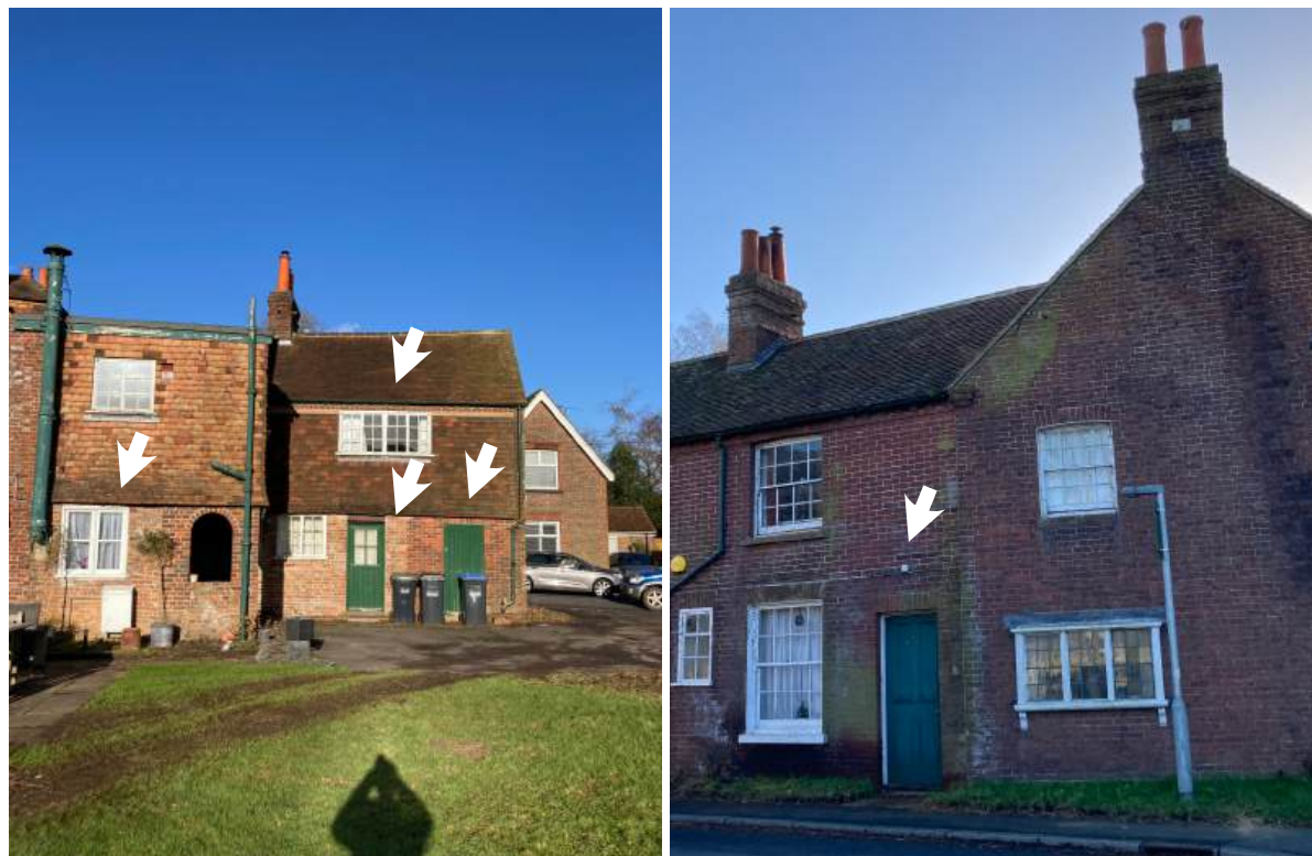
Fenestration to be altered (left) and former surgery door to be blocked and retained (right).
