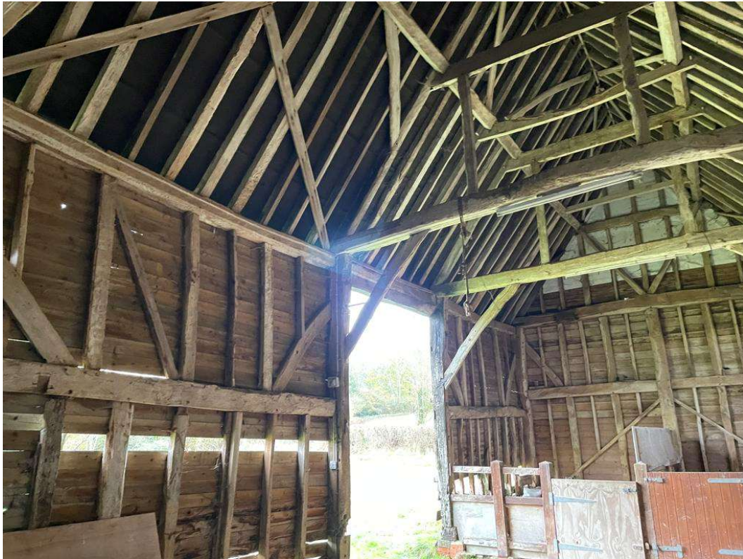
View on front wall of main barn showing posts, tie beams, queen posts and purlins
