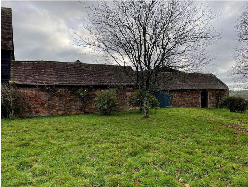
View on brick barns adjoining main timber barn
