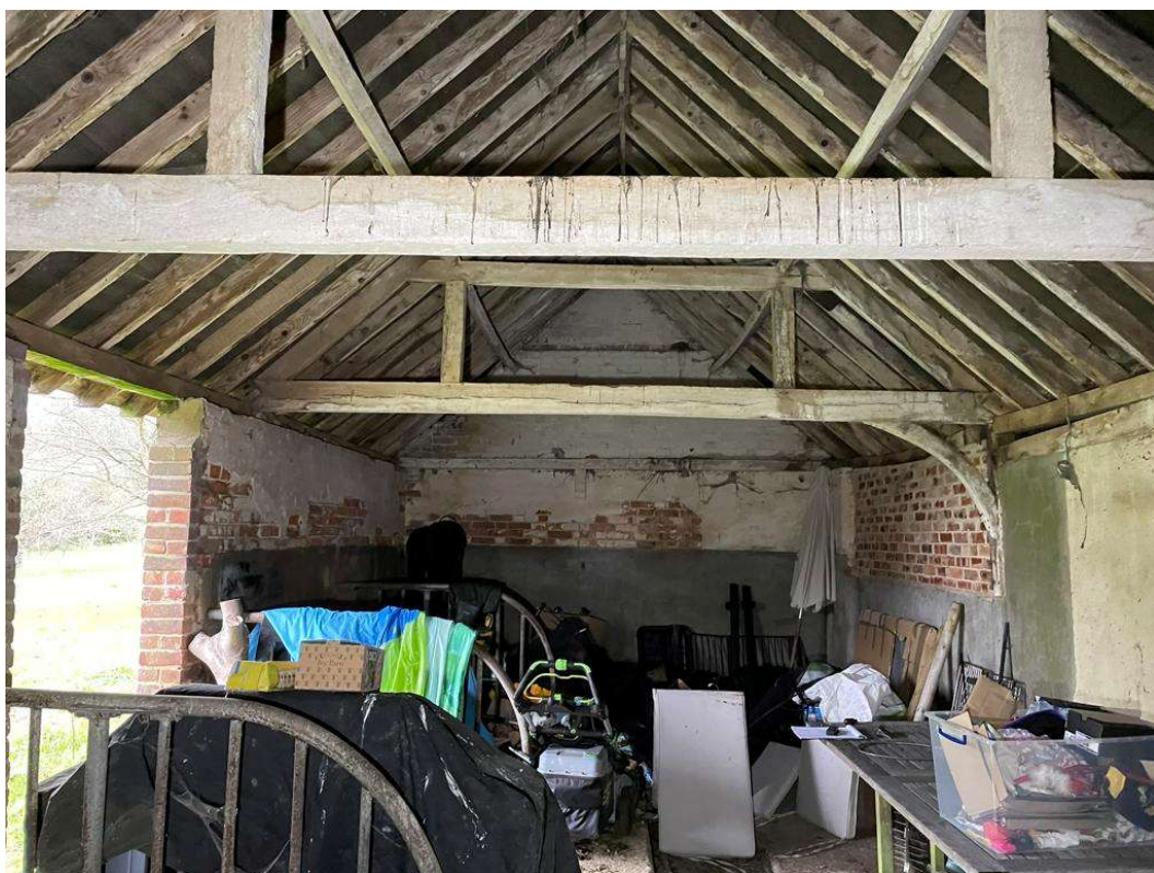
View on roof structure of southernmost barn showing structure as adjoining barn
