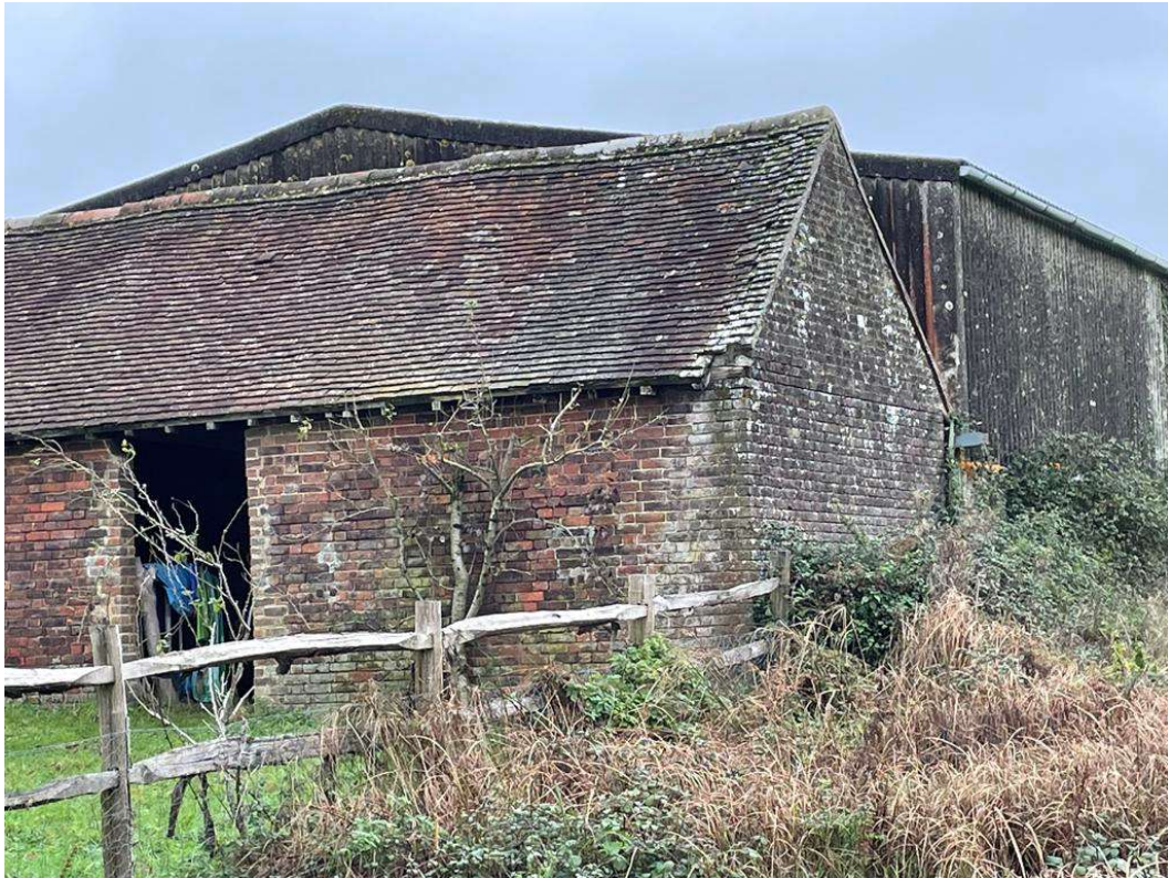
View on southern end of southmost barn
