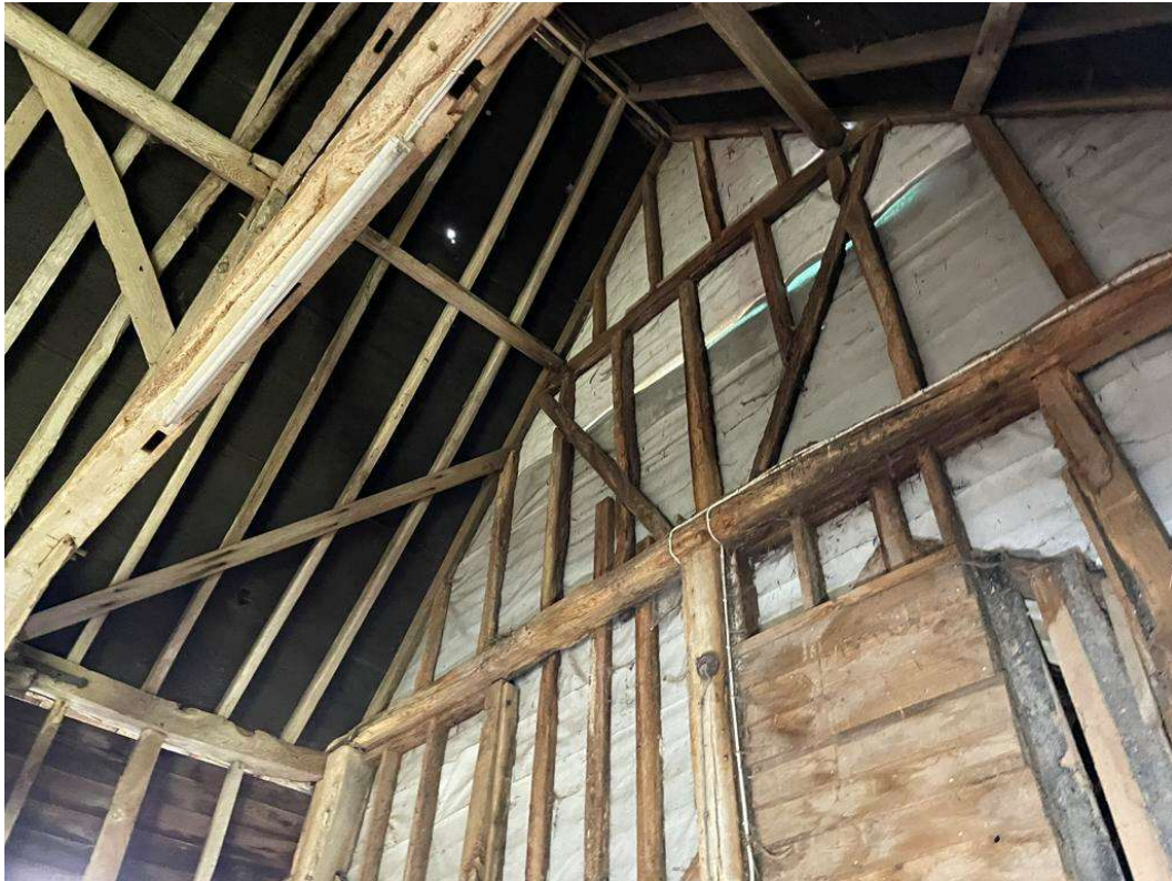
View on main barn gable end showing tie beam and gable framing
