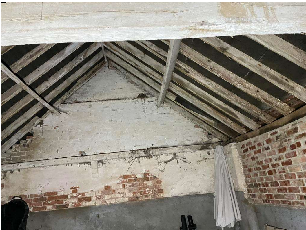
View on gable wall between brick barns
