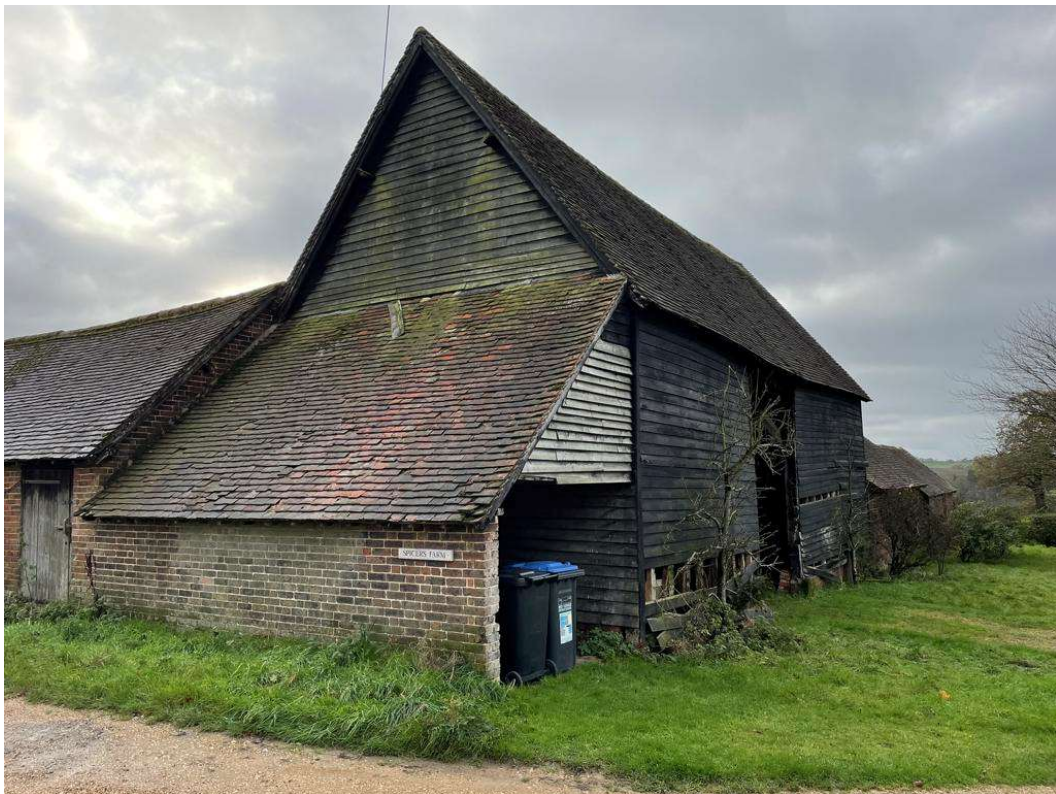
View on lean-to structure to left end of main barn
