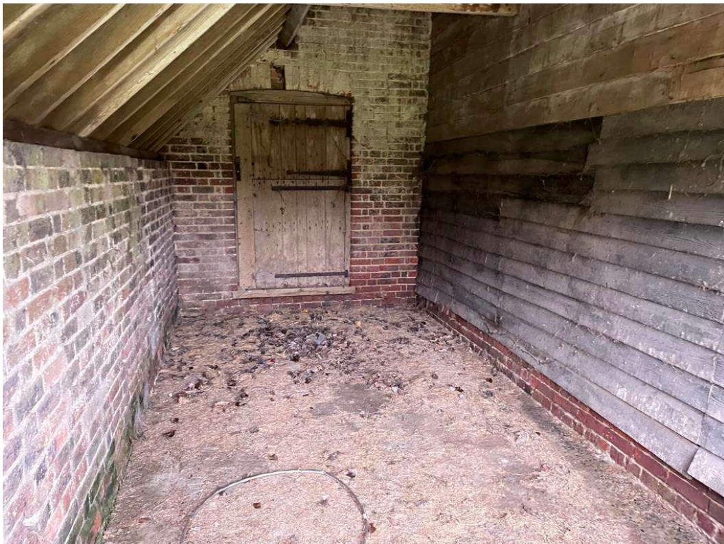
View inside of lean-to building to left of main barn
