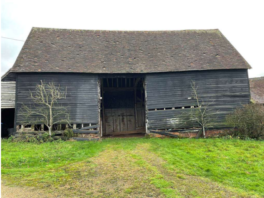
View on front of main barn showing brickwork plinth and timber weatherboarding
