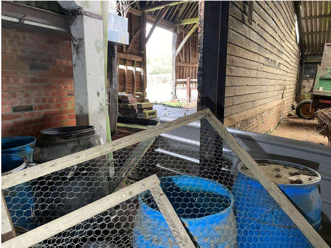
View on rear right corner of main barn from concrete barn showing stagger and brickwork wall of barn
