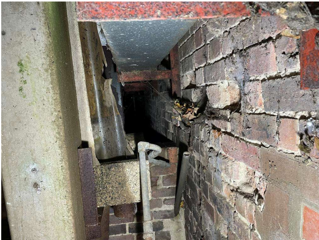
View on underside of valley gutter and rear wall of brickwork barns
