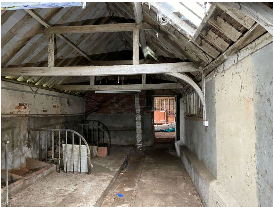
View on barns showing roof trusses, purlins and rafters
