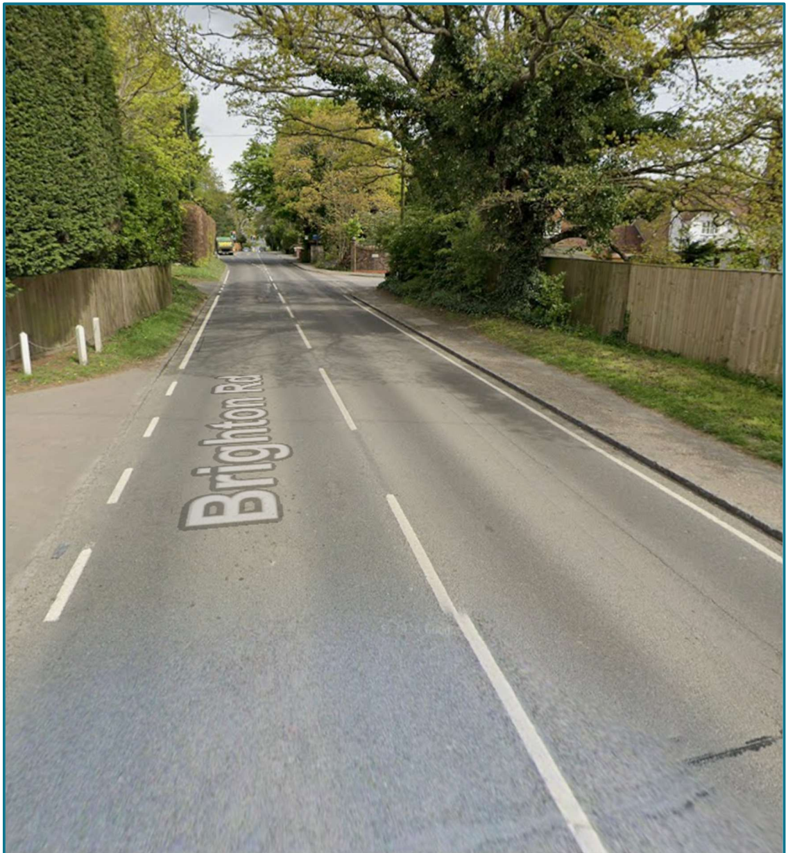
Figure 3.4 – Brighton Road (Northbound)
