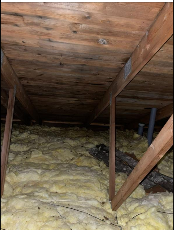
Photograph 4: Loft space with fibreglass insulation.
