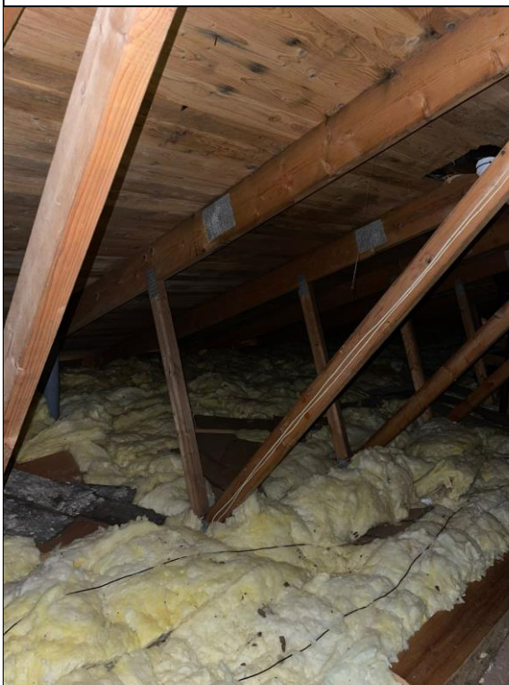
Photograph 3: Loft space with fibreglass insulation.
