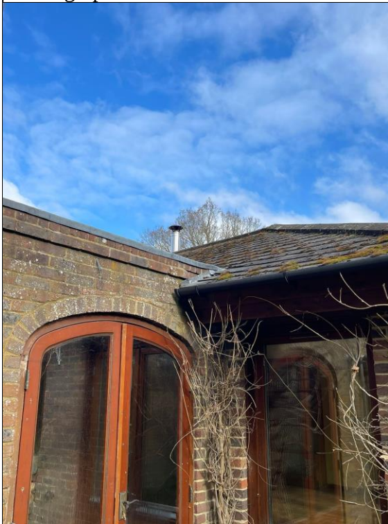
Photograph 11: No visible gaps under roof tiles.
