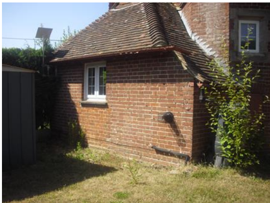
Extension on South Elevation.
