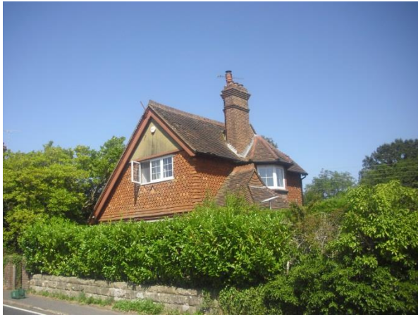
View from London Road looking North East.
