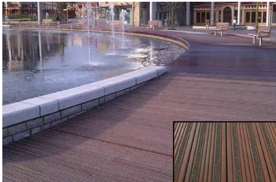
Hardwood decking with anti-slip strips - to platform access.
