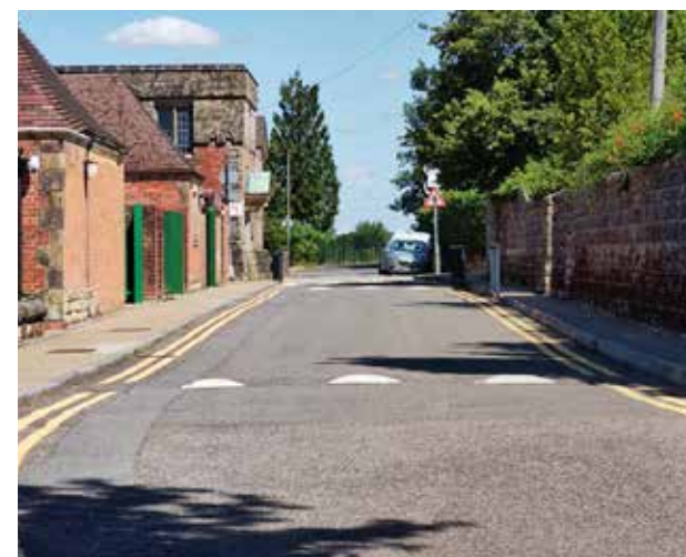
Photograph I - View of the vehicular exit link.
