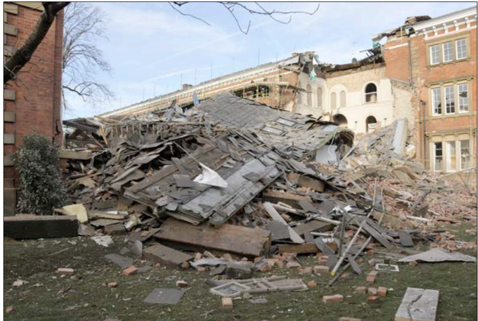
Figure 1 Aftermath of a gas explosion, following damage to an underground gas service pipe
