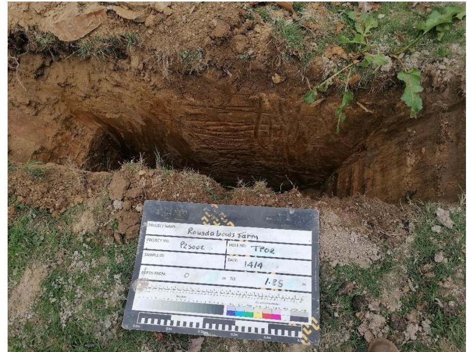
TP02 trial pit
