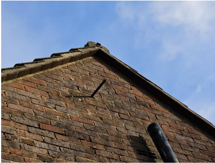
Photograph 2: Example of the gable wall showing fully mortared tile runs and mortar sealed wall top to tile junction
