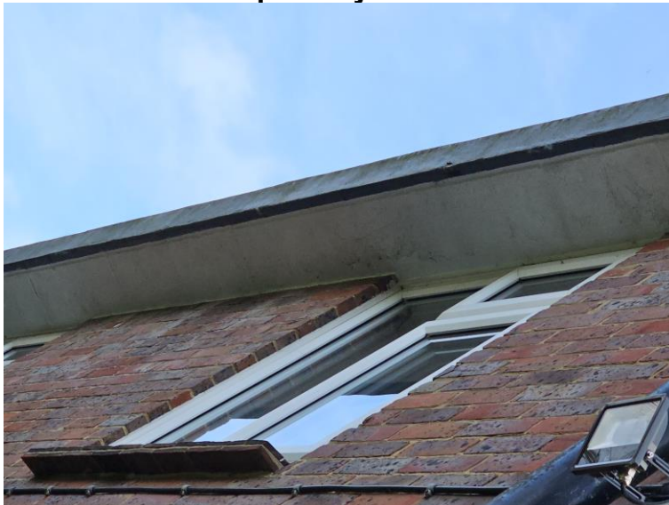
Photograph 3: Mastic sealed wall to soffit box junction
