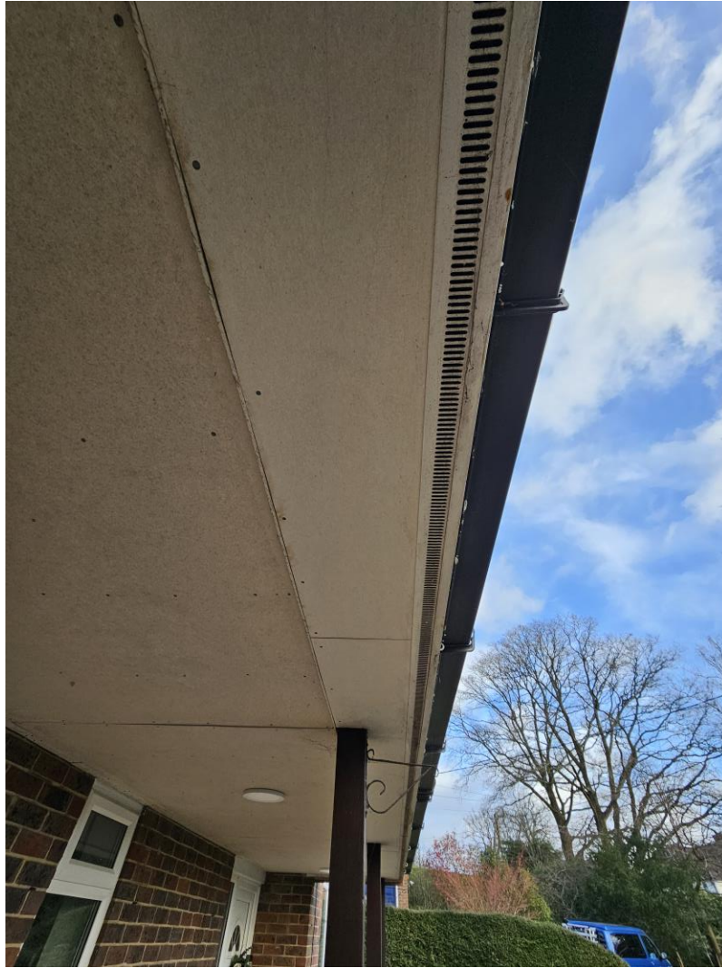
Photograph 4: Meshed vent to lower level and garage
