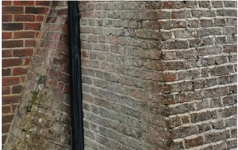
Brickwork to match existing
