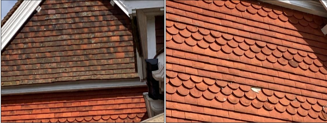
Photographs 2a (left) and 2b (right). 2a) View of hanging tiles located to the southern aspect of the property with some signs of lifted and damaged tiles visible. 2b) View of hanging tiles located on the property with clear signs of damage, lifting and missing tiles.
