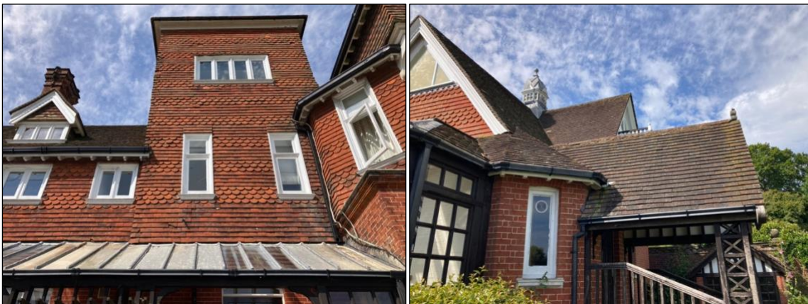
Photographs 4a (left) and 4b (right). 4a) View of the former tower block located to the centre left of the image, image taken from the eastern aspect of the property, clear signs of damage to hanging tiles noted included lifted and missing tiles throughout image. 4b) View of the northern aspect of the property with the image taken from the eastern aspect, some signs of damaged roofing tiles noted to these aspects.
