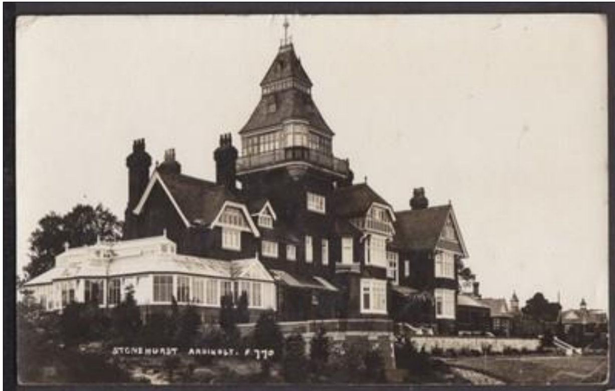
Figure 3. Historic view of Stonehurst Main house with view of the tower. Image produced courtesy of Ian Adam Smith Architects.
