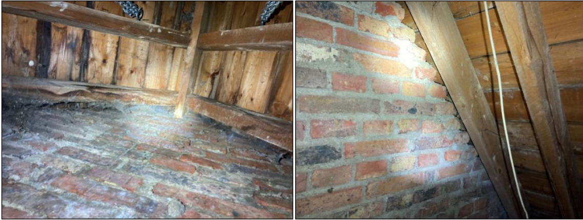
Photographs 8a (left) and 8b (right). 8a) View of the rear wall with gaps to the exterior/roof lining noted to the top of image. The image also illustrates the ridge beam and rafters that are typical throughout the loft space that can act as roosting opportunities for cavity dwelling bat species. 8b) View of the gaps to lining as shown in photograph 8a from approximately 0.5m away.
