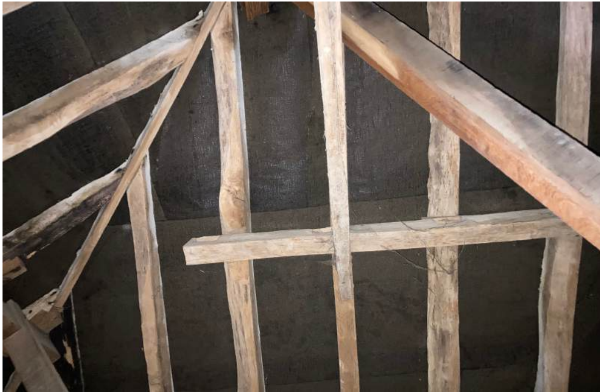
Roof structure over rear wings.
