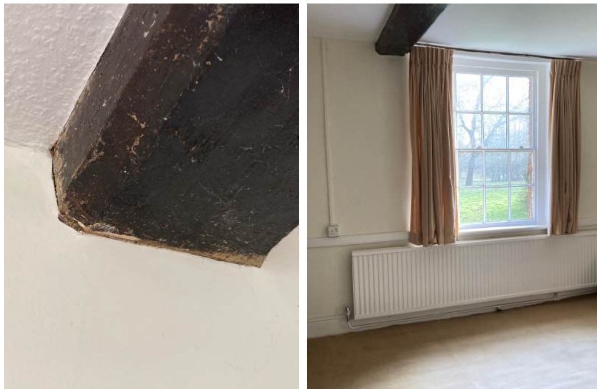
Detail of bridging beam displaying run-out chamfer stop and awkward location of later inserted sash in relationship with earlier bridging beam.
