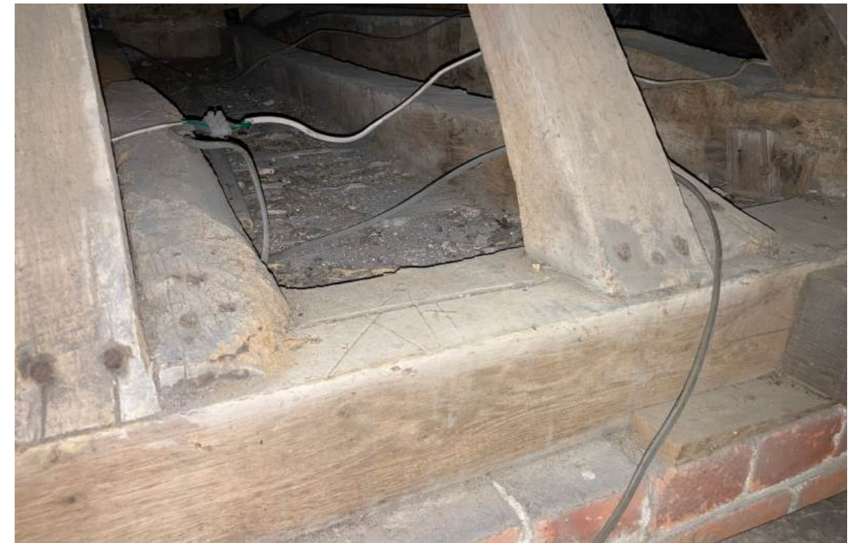
Detail of roof structure over main range. Note the presence of carpenter marks.
