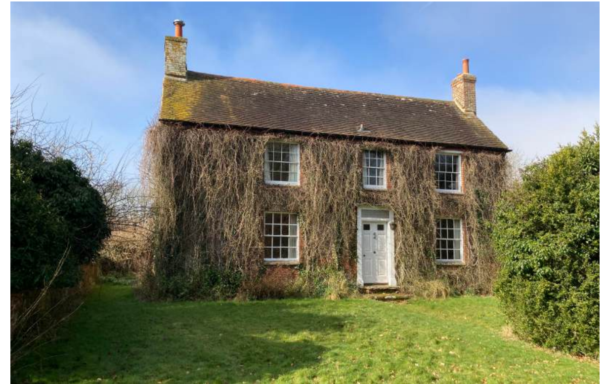
East (front) elevation of the farmhouse.
