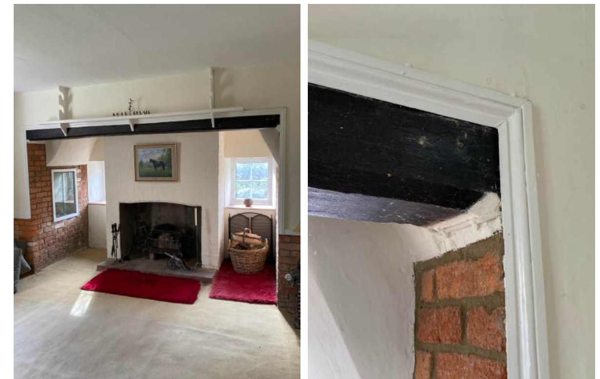
Original late C17/early C18 inglenook and detail of run-out chamfer stop decorating the lintel.
