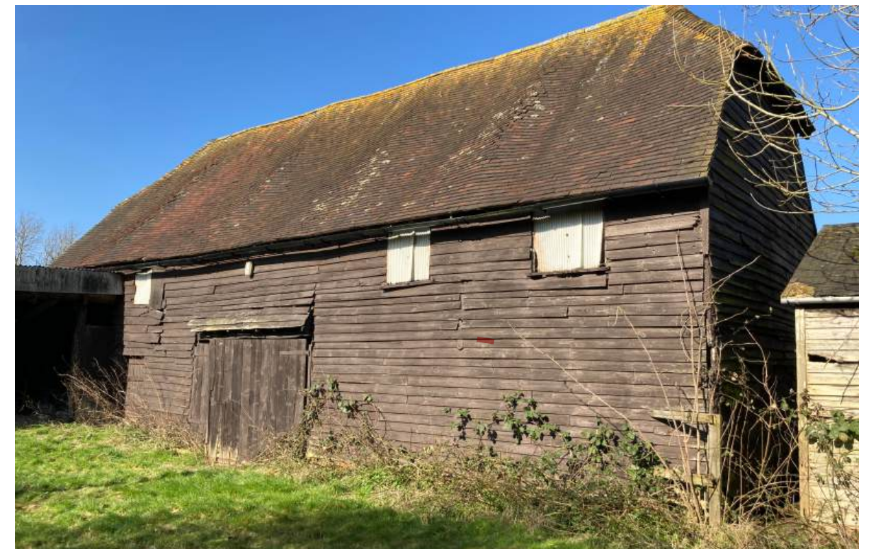
Grade II Listed barn to the south of West House Farmhouse
