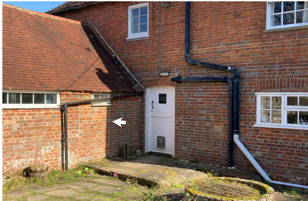
Location of new opening. Note the evidence of previous alterations.
