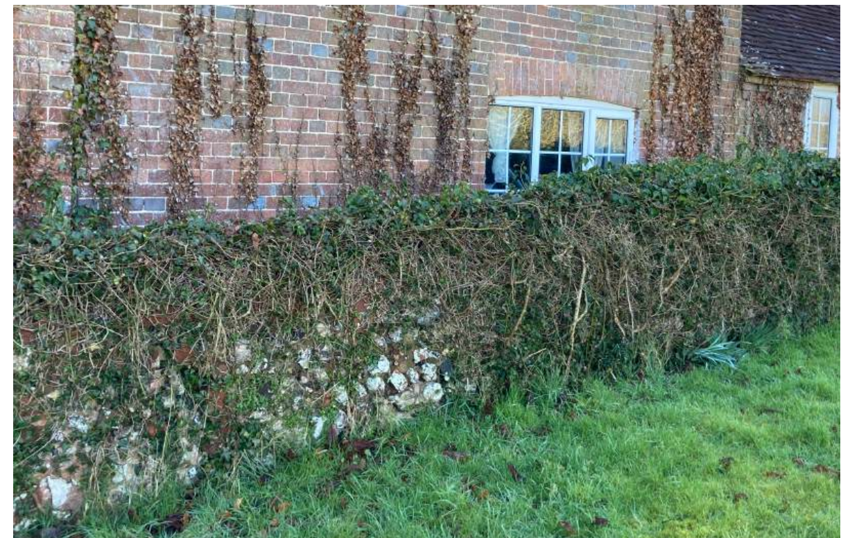
Existing window to be converted into a doorway.
