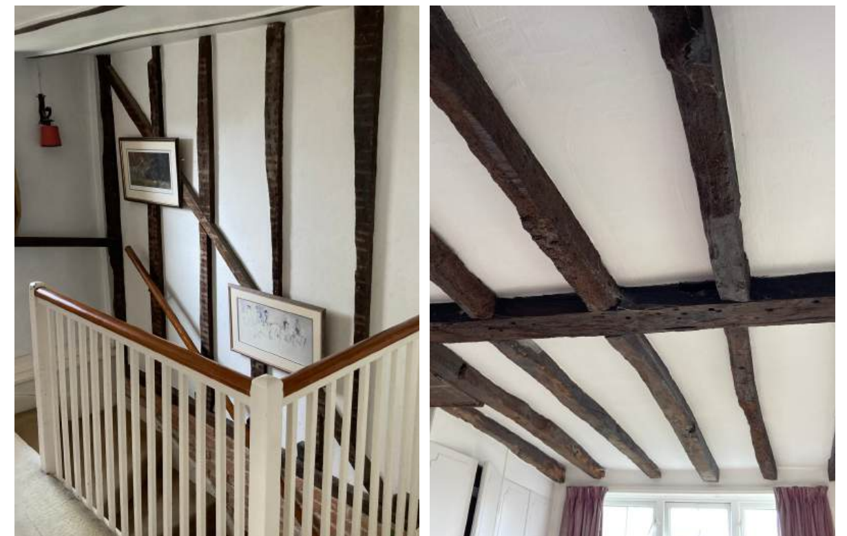
Timber-framed partition and exposed joists and bridging beam within rear wings.
