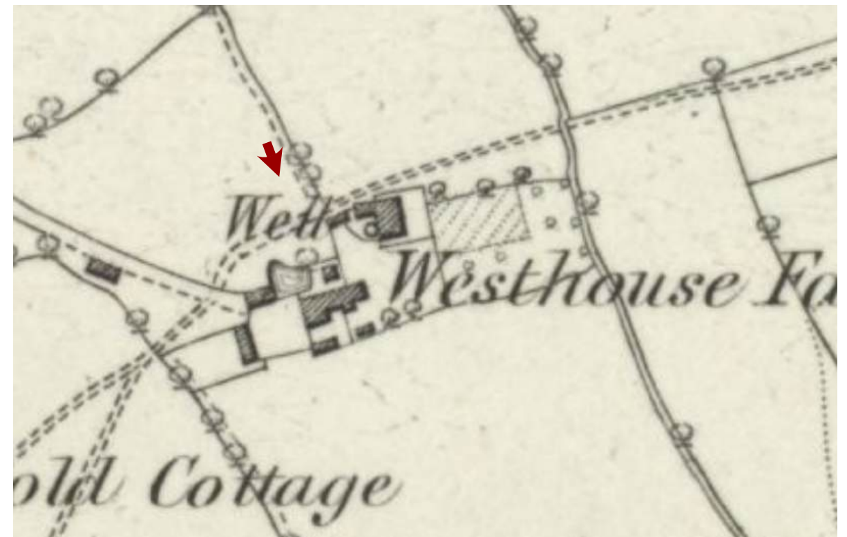
Detail of Ordnance Survey showing Westhouse Farm, 1874 (National Library of Scotland).
