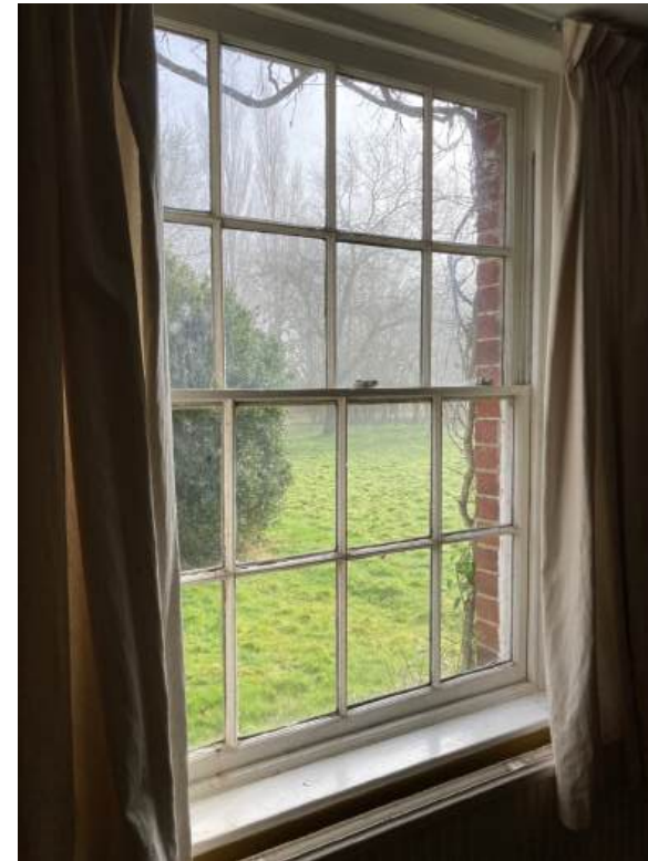
Example of surviving Georgian sash and panelled door.
