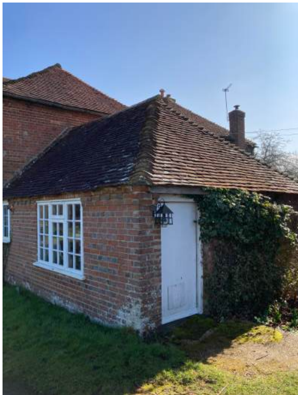
Former brewhouse/washhouse. Note the ventilation windows.
