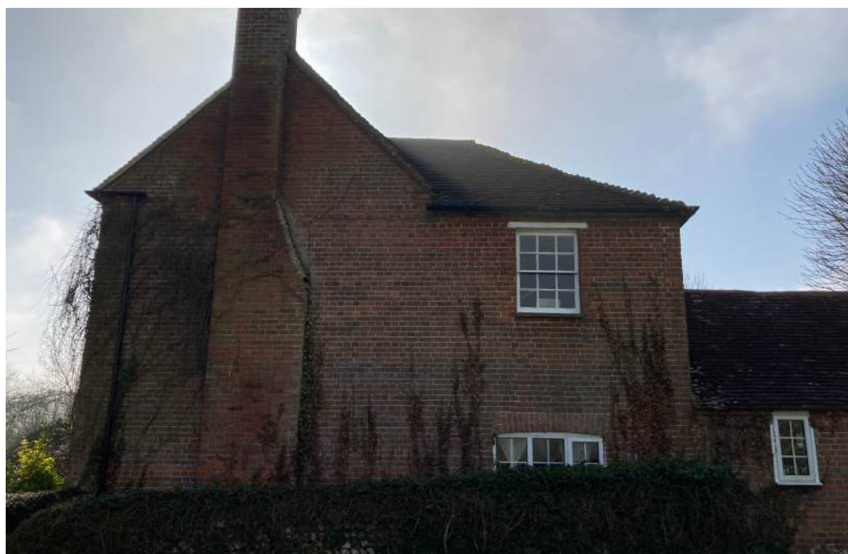
North elevation of the farmhouse.
