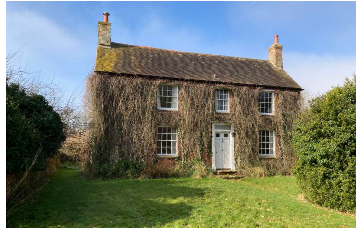
Grade II Listed West House Farmhouse
