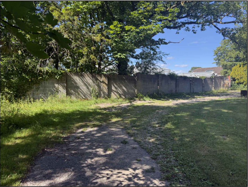
EXISTING NORTHERN BOUNDARY WALL
