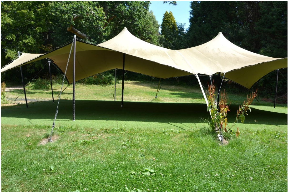
Figure 17: Shot 2 - closer view of the existing tent structure and concrete base, looking E.
