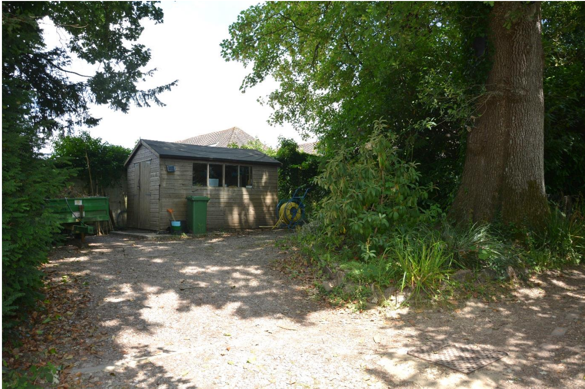
Figure 30: Shot 15 - view of the existing garden shed on the northern side of the northern path through the site, looking NE.
