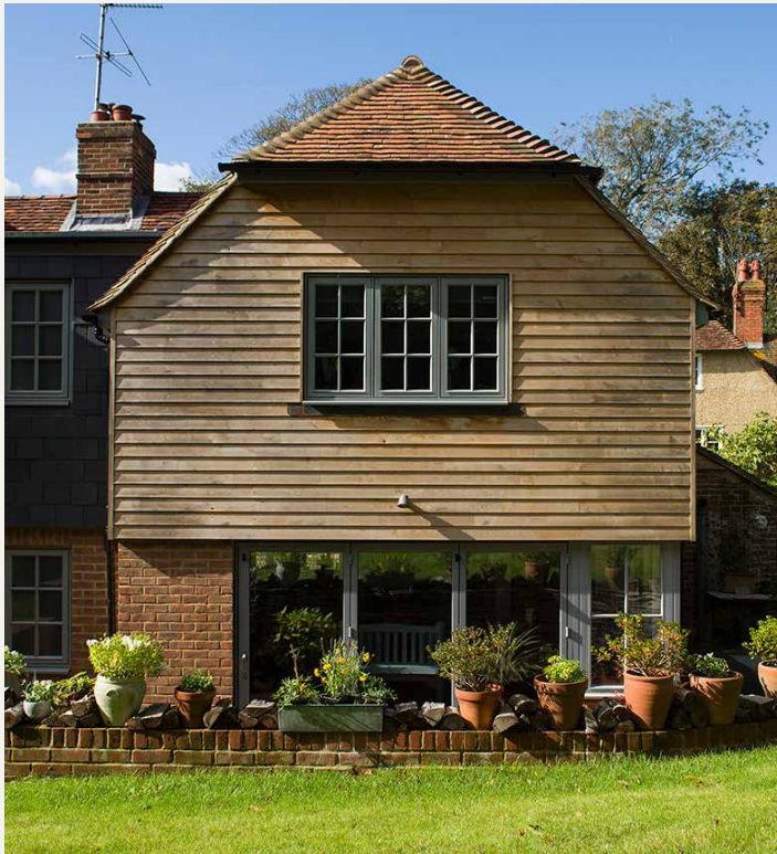
Similar brick and timber cladding arrangement.
