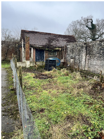
IM01 - View from garden looking west
