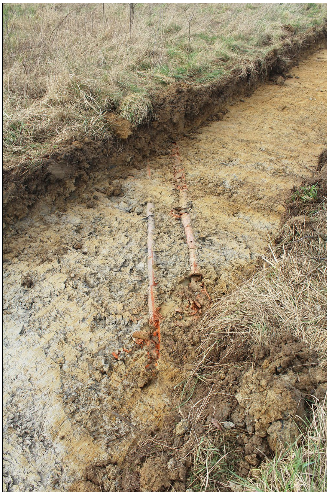
Figure 6 The pair of parallel land drains in Trench 4, looking west
