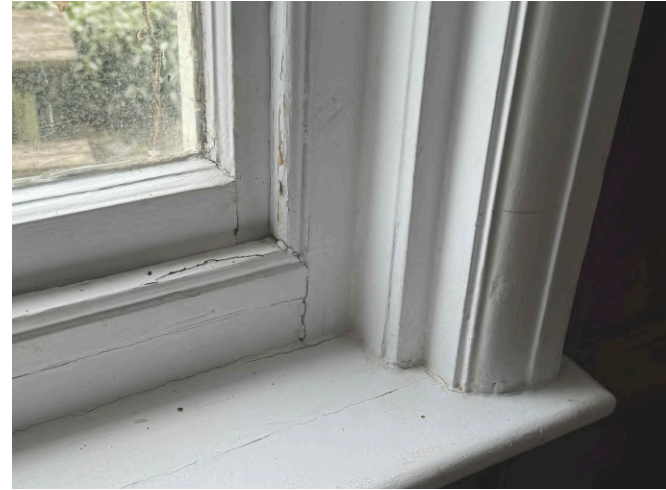
Typical sash window
