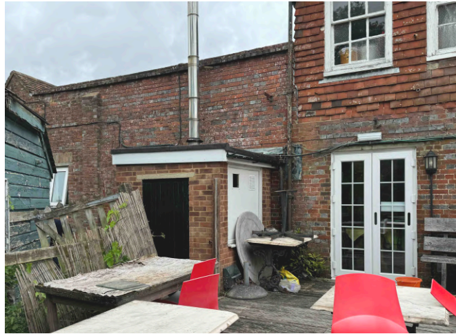
South Elevation (Stables and farmhouse junction)
