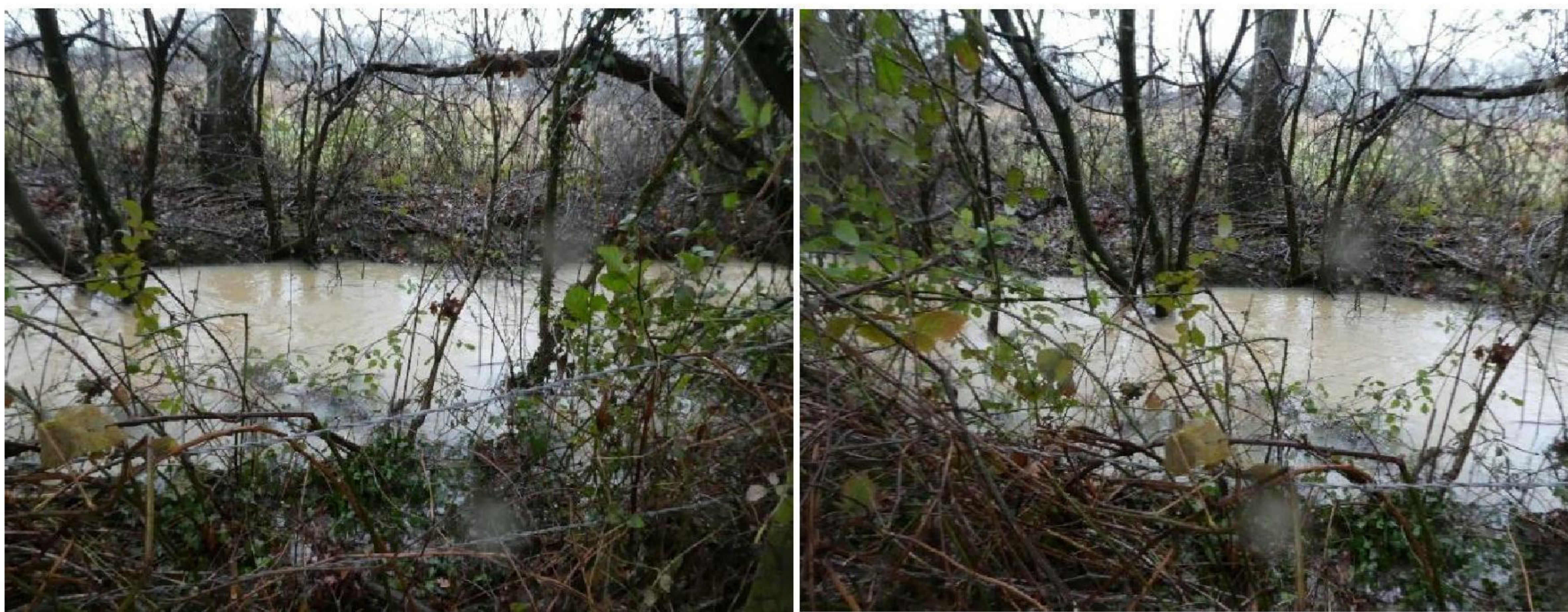
Photographs taken 27/01/2026 showing that the watercourse had reached its full capacity along the whole of its route along the site's western boundary
