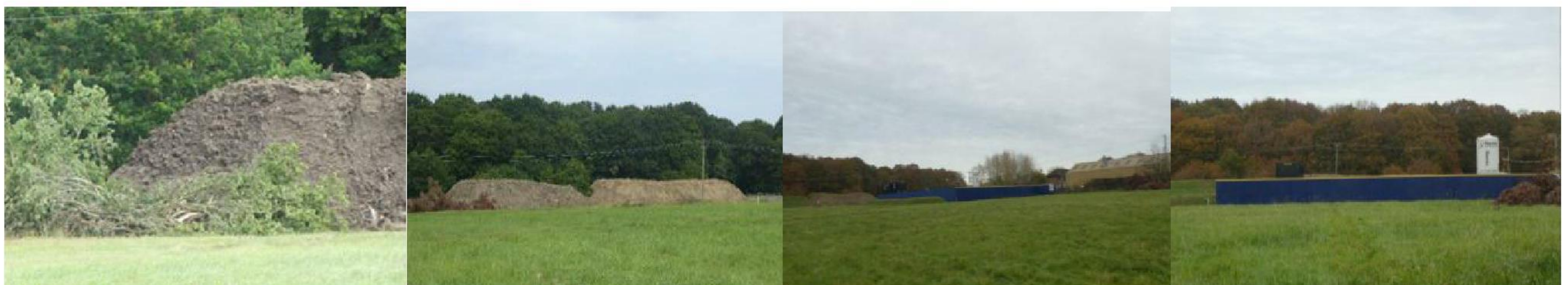
Photographs of the spoil heaps started in June 2024 and the compound built soon afterwards
