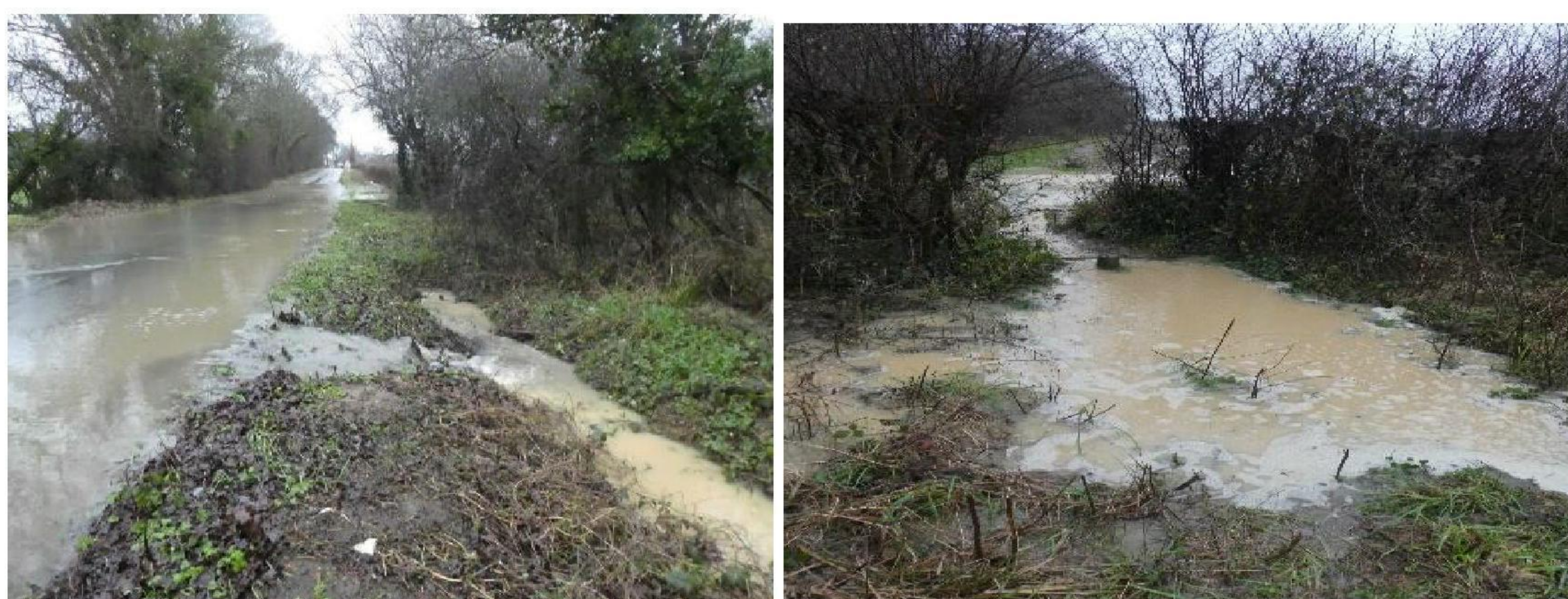
Photographs taken 05/01/2025. Left Reeds Lane flooded at the point that the new footpath from the site will exit onto it. Right, the flooded entrance to the southern side PROW 3A1 with flood water pouring down through it onto Reeds Lane as the verge ditches can not contain it
