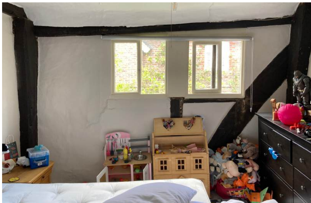
First-floor rear room wall to be insulated.
