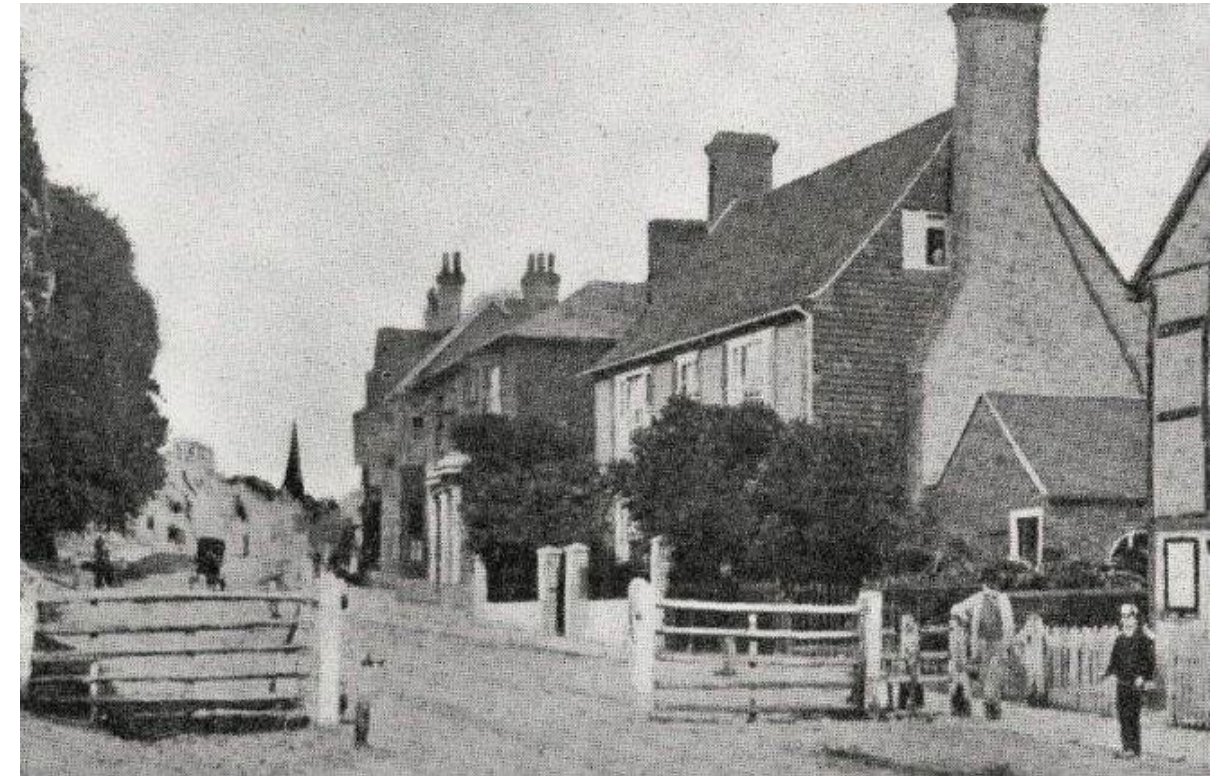
The toll gates with The Toll House to the right (looking north), c.1880.
