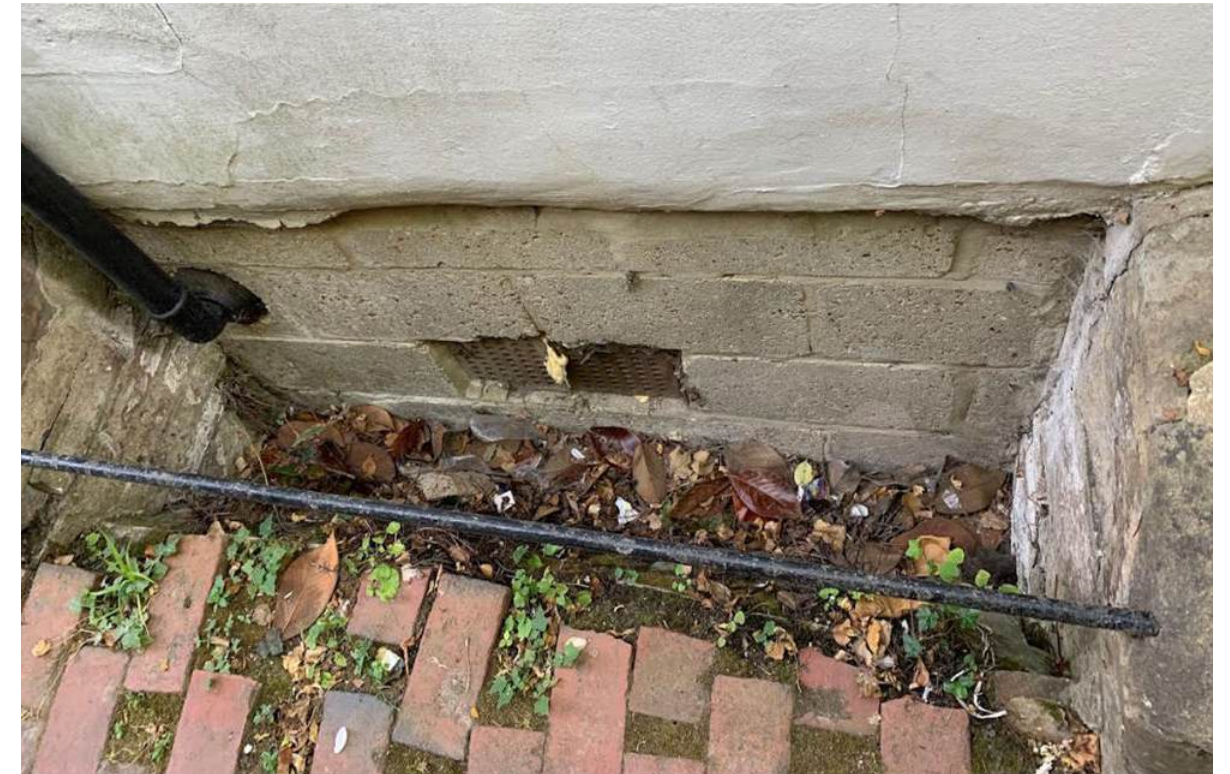
Basement window to be reinstated.
