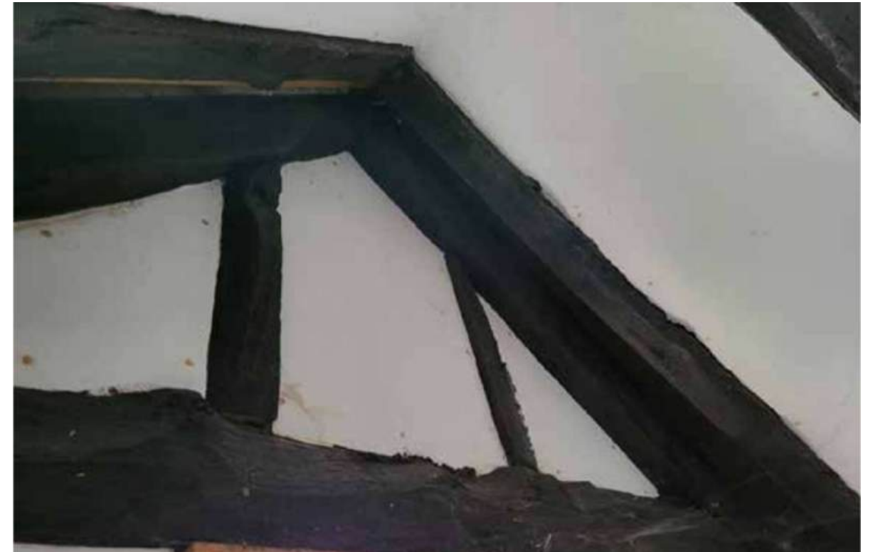
West gable to be insulated.
