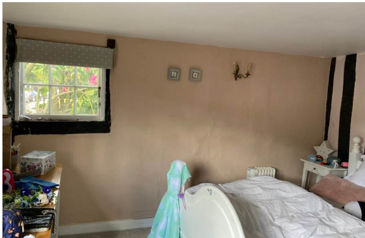
First-floor front room wall to be insulated.
