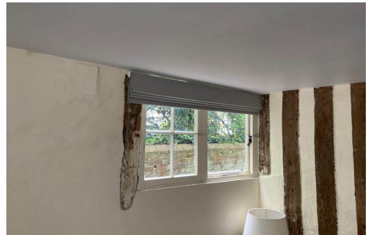
Ground floor front room wall to be insulated.
