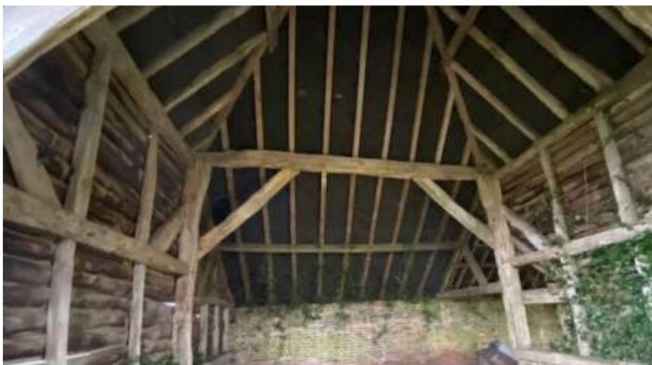
Internal view of the tall barn showing the roof structure
