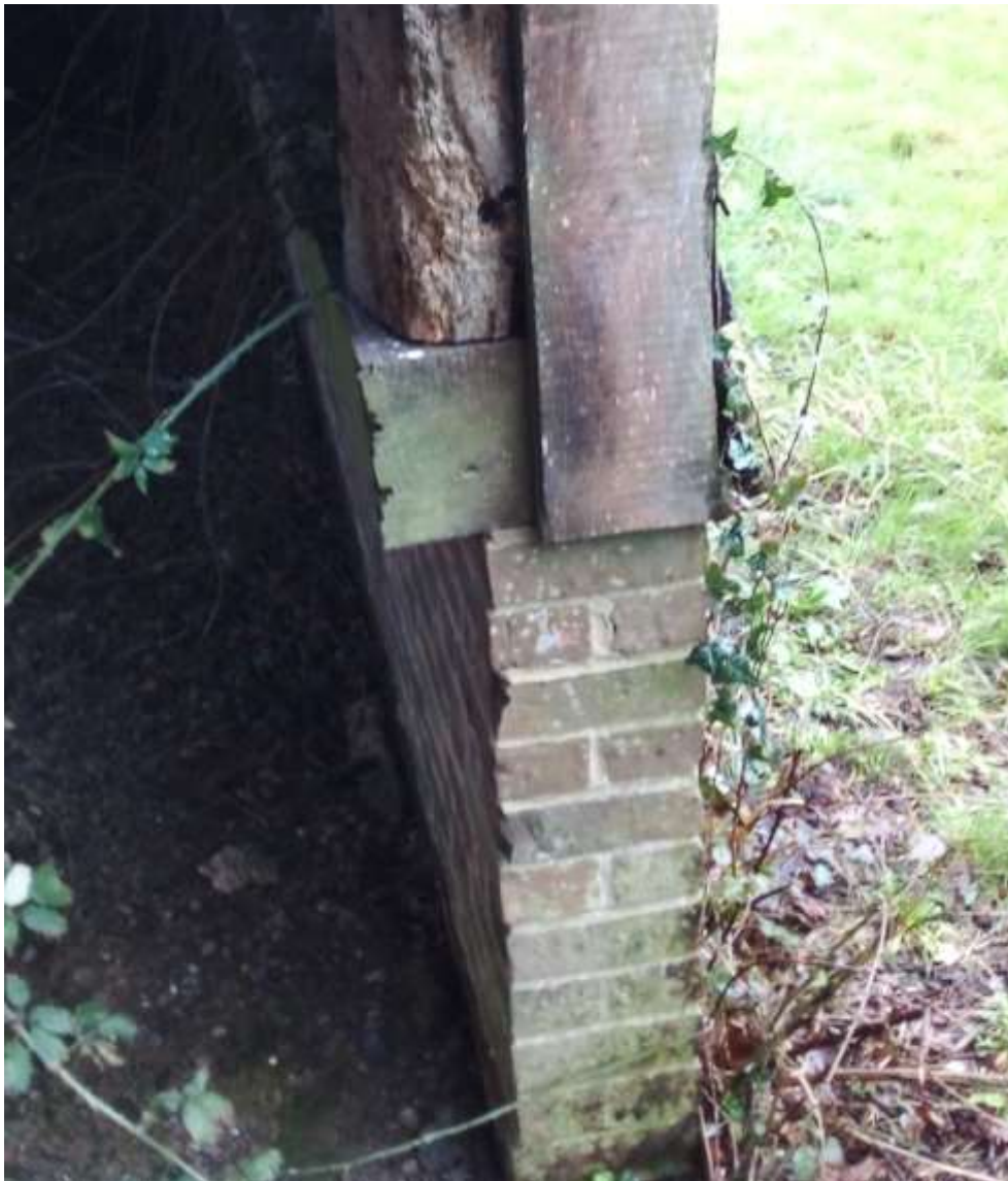
The dwarf walls, sole plates and oak posts are all in good condition
